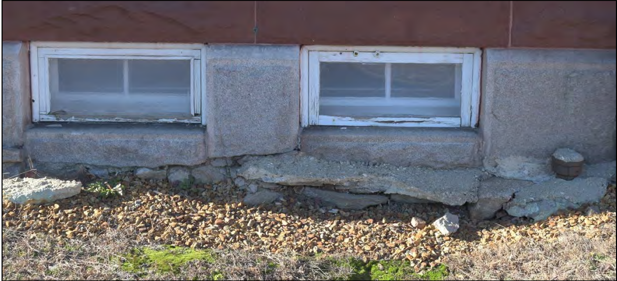
Figure 64: Remains of historic concrete apron at east elevation of main block with plugged drainpipe at right
