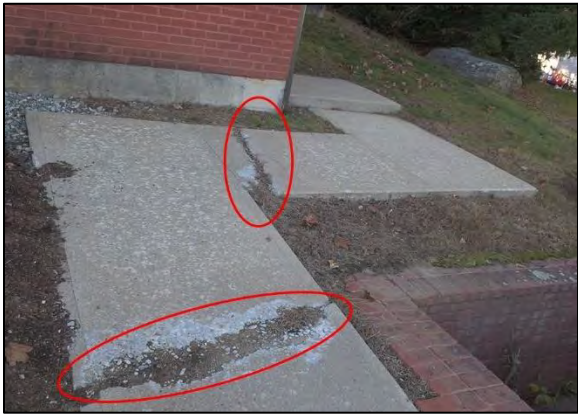
Figure 68: Cracked modern concrete path
