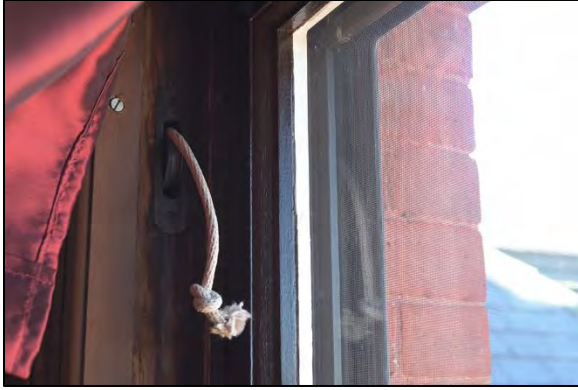
Figure 80: Broken sash cord of 1895 historic window
