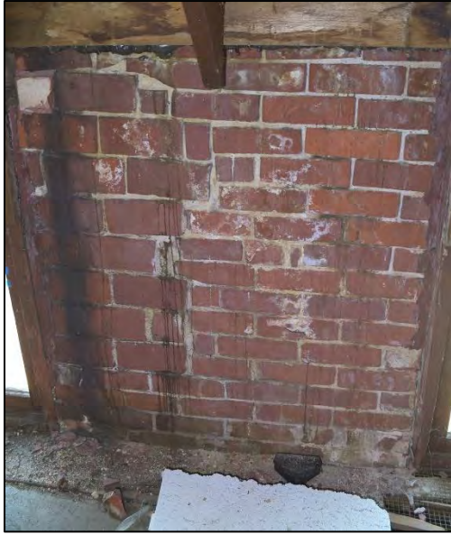
Figure 76: Stained and spalled brick of west chimney, photographed from attic
