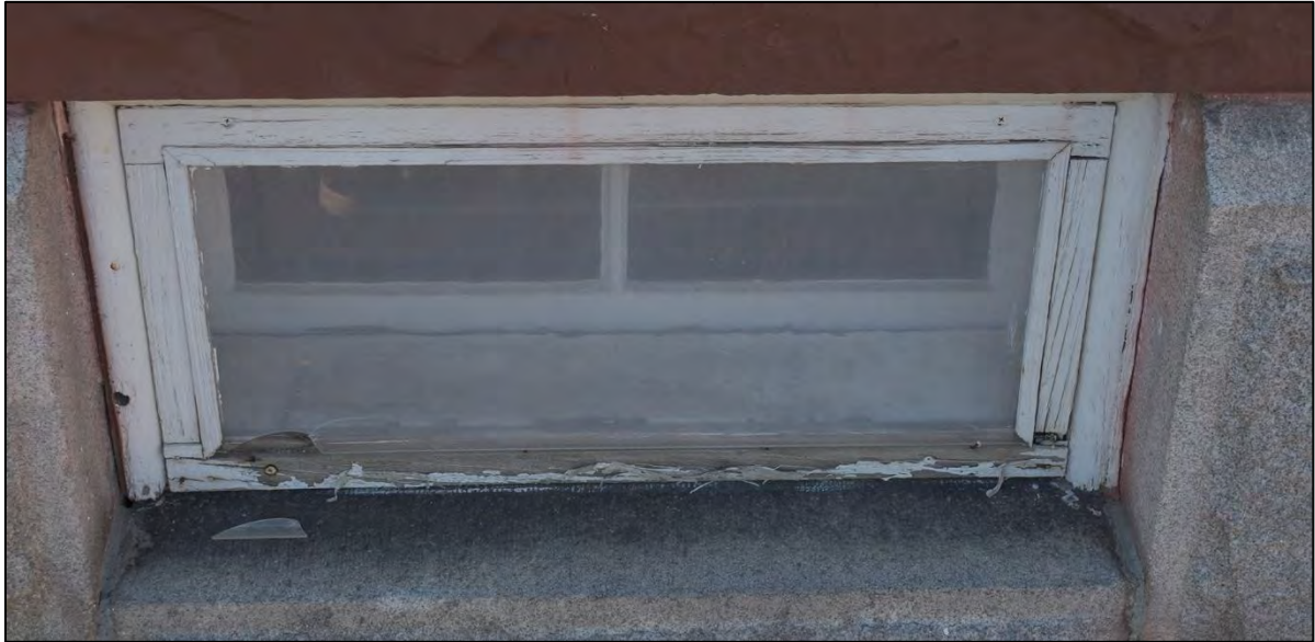
Figure 79: Damaged basement storm window at east side of main block
