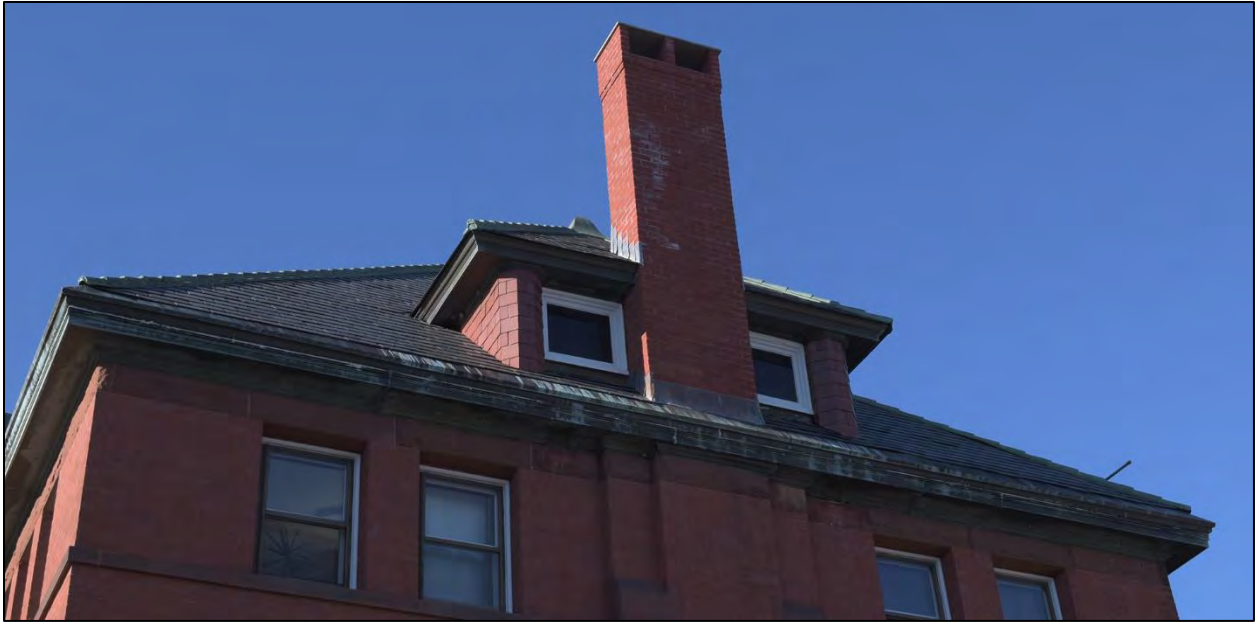
Figure 21: Hipped dormer with integrated end chimney
