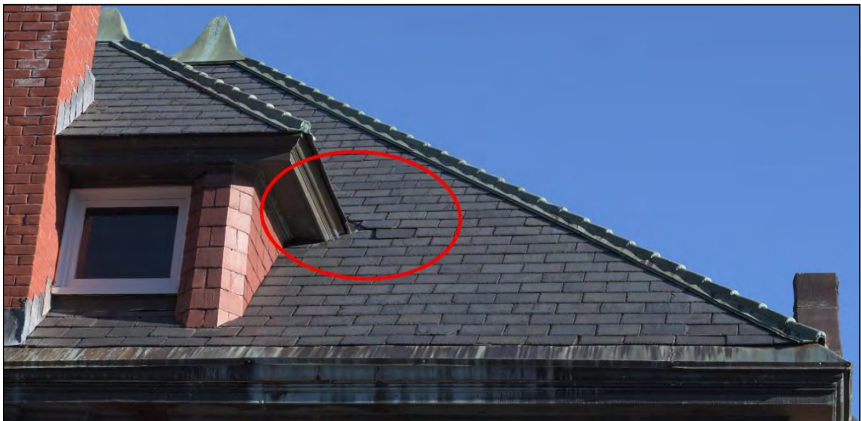
Figure 71: Damaged slates at west roof slope
