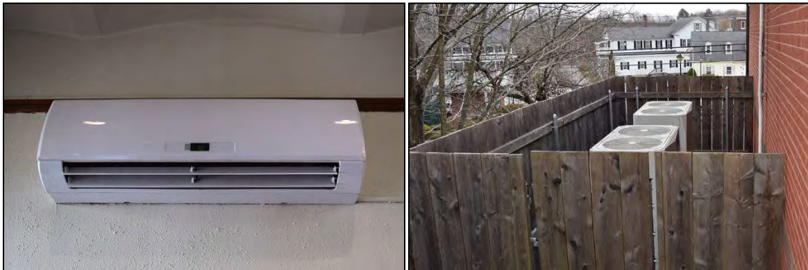
Figures 92 & 93: Typical VRF head unit (left) in historic building and condenser outside modern addition (right) (Photographs courtesy Brian Gallien)
