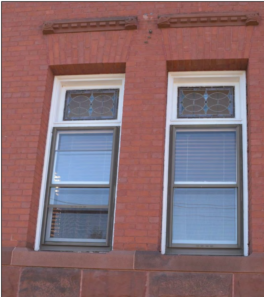
Figure 78: Typical first-floor windows with operable one-over-one sash beneath a fixed stained-glass transom
