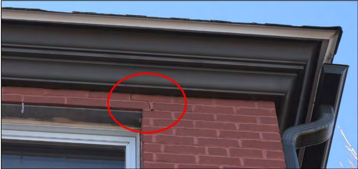
Figure 74: Small crack in exterior masonry at southeast corner of main block
