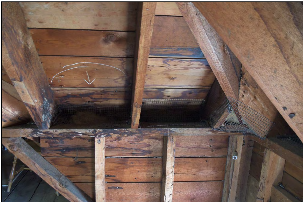
Figure 73: Water-staining at south side of west attic dormer (Note: hardware cloth at eave to prevent pests)
