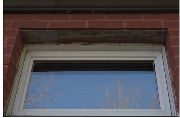
Figure 81: Rusty header and failing caulking at 1989 window
