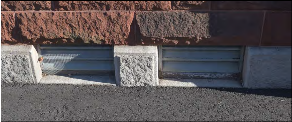
Figure 67: West side of main block, showing asphalt poured directly against basement window sills
