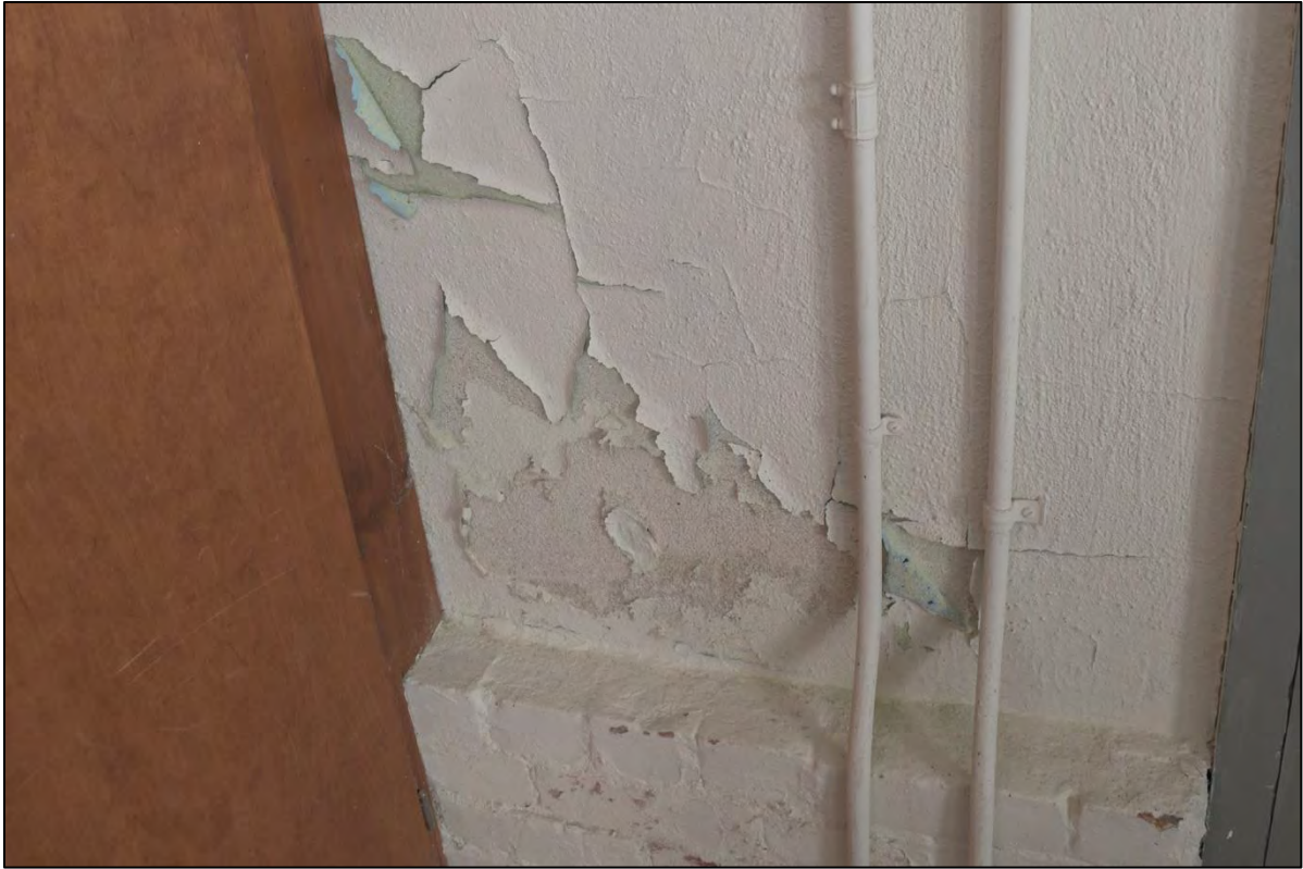
Figure 88: Peeling paint at southeast corner of first-floor landing in historic stair
