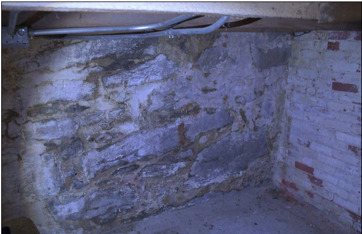
Figure 85: Discolored mortar at rubble stone foundation (west wall) inside of historic stair. Note: traces of white sealant was added to these walls in 1975-1976.
