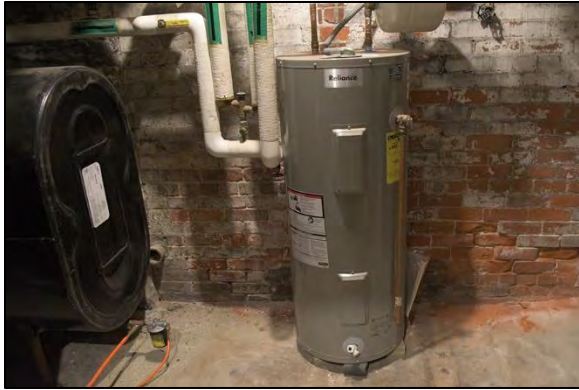
Figure 98: Hot water tank
