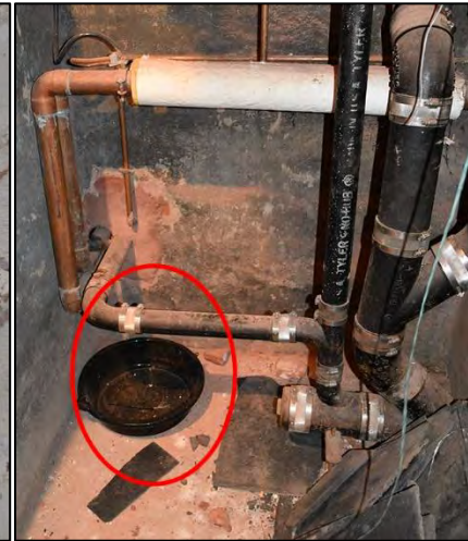
Figure 97: Actively leaking pipe
