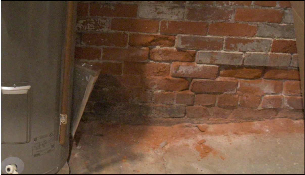
Figure 86: Spalling brick at north wall of mechanical room
