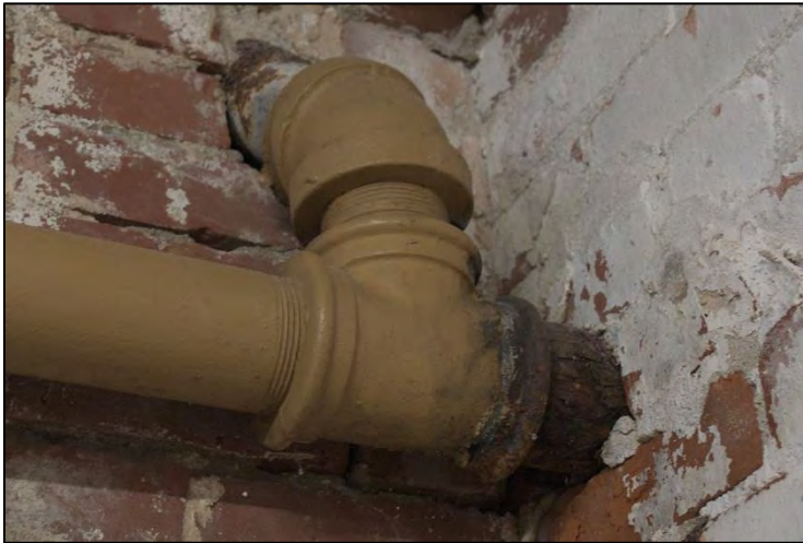
Figure 96: Extremely rusted cast-iron pipe
