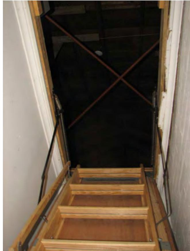
Attic drop down ladder has large air gaps, is uninsulated, and is also rickety.
