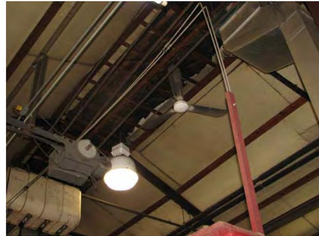
Ceiling fans used to try to force warm air back down with little effect.
