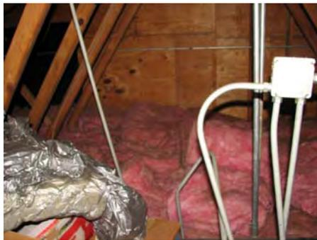
A thorough air sealing of this ceiling is necessary to realize meaningful heat loss reductions. In this case, with so many ceiling penetrations and evidence of moisture, removing all fiberglass and spraying a 1-2" skim layer of closed cell foam over the entire assembly (dry wall, strapping, and joists), will create a
