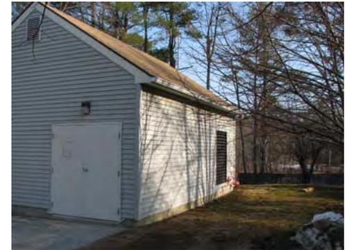
Approx 20 x 24 shed with 2x4 framed walls; 3.5” fg batts. 10’2 ceilings and roof vented with continuous soffit and gable end vents.
