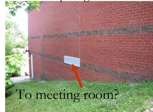
Outside fresh air (all year) drawn into three fan coil wall units. These openings were not sealed for the blower door test so are part of the total 12sf hole in the wall!
