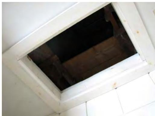
This attic hatch is left open so that conditioned air can keep pipes located in this attic from freezing. This is perhaps the greatest single source of heat loss in the building. Since IR indicates that there are anomalies throughout the ceiling and that comprehensive air sealing
