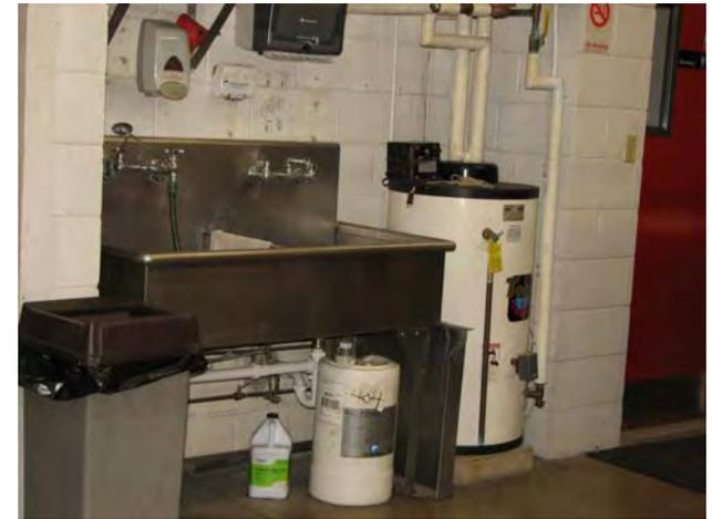
Site visit: July 25<sup>th</sup> 2010, 8am. 76 degrees and humid. Boiler comes on to heat hot water for 15 minutes – boiler room gets to 87°F. Even with 35 gallon heat exchange tank, over 200 gallons oil used to heat water in summer – from cycling 483MMBtu Burnham boiler.
