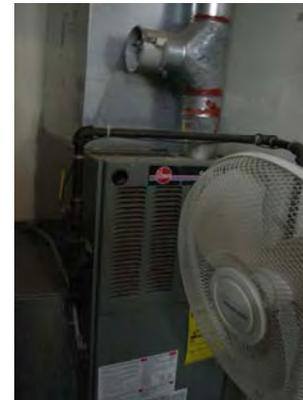
Rheem Criterion II forced hot air furnace – 80% AFUE
