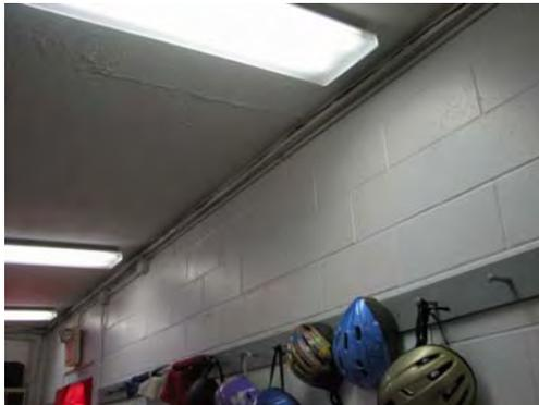
Edges where the walls meet the ceiling, and the slab, are sources of heat loss and personal discomfort.
