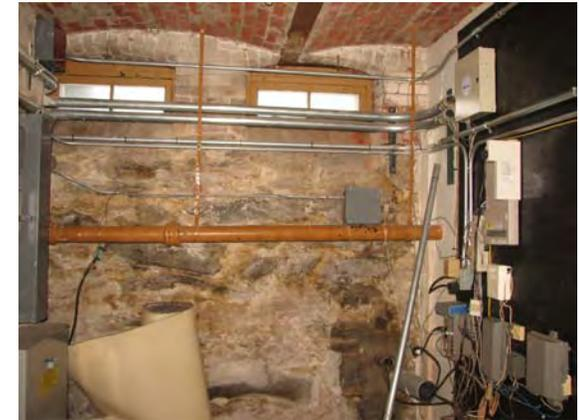
Foundation walls lose a lot of heat, estimated at 6% of envelope heat loss in this library. That's equal to the conductive losses from the 1990 addition!
