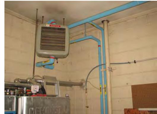
Two thermostatically controlled hot water Modines – office and garage.
