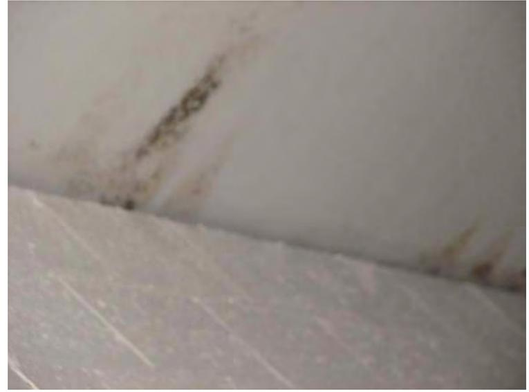
Indications of air transported moisture at transition of roof and wall.
