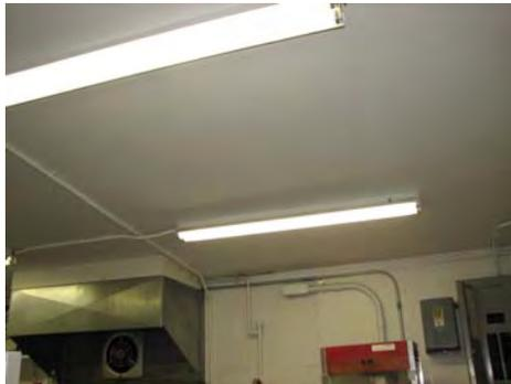
Insulation values above the ceiling are not known, but it appears that there may be some level of insulation over the framing, as if blown or a second layer of batts had been added. A guesstimate for the ceiling assembly is between R14-16.
