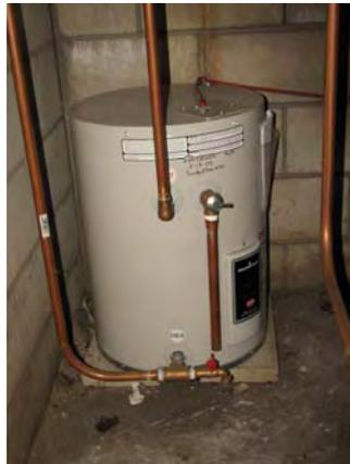
Bradford and White Indirect water heater, installed in 2009
