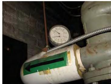
Water temperature can be adjusted for shoulder seasons, though true modulating boilers with outdoor reset sensors would be more efficient.
