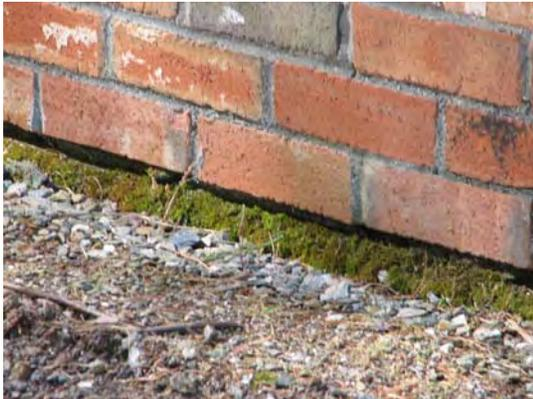
It appears that there is mortar between the brick veneer and slab foundation, yet no evidence of weep holes from the drainage plane. The moss may be a result of wicked moisture's downward flow? Or surface drainage towards, not away, from the building?
