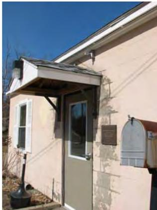
A 40' x 100' concrete block building built in 1964, with a 22'x28' frame addition in the back. The bay doors face southeast, potentially offering an excellent location for a roof mounted PV array.
