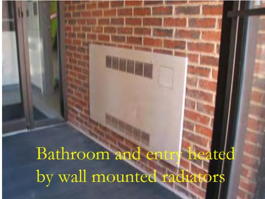
Bathroom and entry heated by wall mounted radiators
