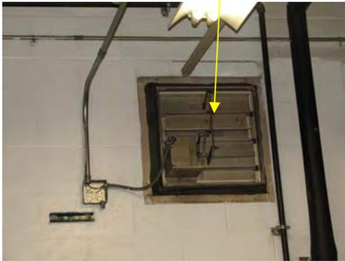
Combustion make up air mechanical vents – wired together
