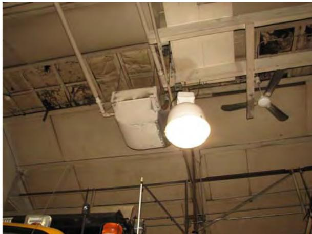
Four large Mercury Halide lights in addition to 8 foot T12 fluorescent lamps.
