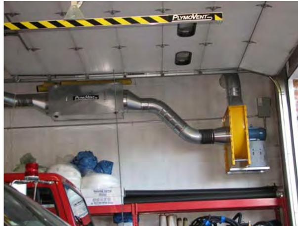
Code compliant Plymovent Vehicle Exhaust
