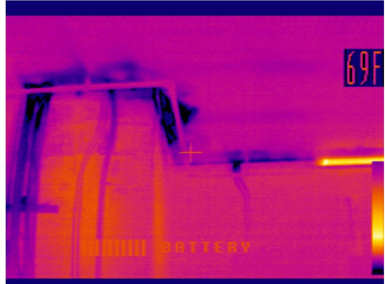
Damage from past water leakage are a constant source of air leakage and heat loss.
