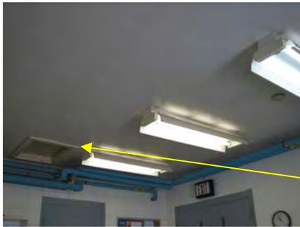
Attic hatch needs air sealing and an insulated cover.
