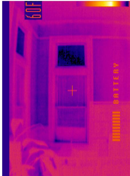
Recommend interior, thermal pane, air sealed, storms on all fixed panes, and to consider removable interior storms for the operable sashes.
