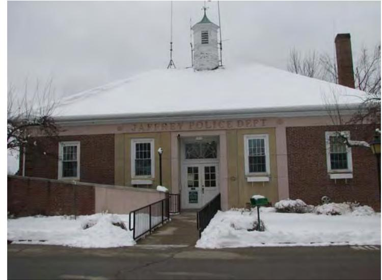
The Police Station is approximately 30'x58', two story, masonry structure built in 1954. Grade slopes on either side, making the lower level at grade on the north facing side, where a single story masonry “sally port” was added side in the mid 90’s. The front faces Main Street and slightly southwest. It has impressive solar collecting roof potential.
