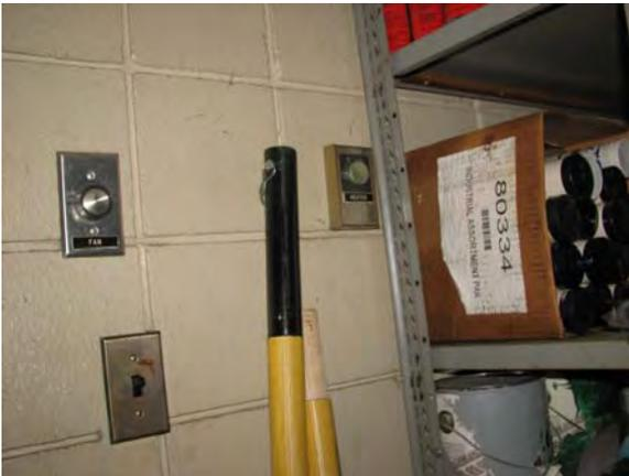
Garage exhaust manually timer operated and without heat recovery
