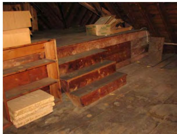
In fact, while adding insulation would also be advised, “simply” establishing a continuous air barrier would make a significant difference to this attic and the library as a whole.
