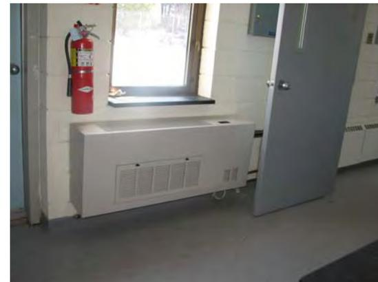
Hot water fan assisted wall heater with fresh air supply.
