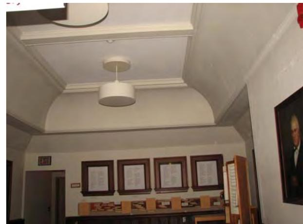
This appears to be a framed section of wall above the stone or brick- and an opportunity to insulate from above. Cellulose or even foam is recommended. Not fiberglass.
