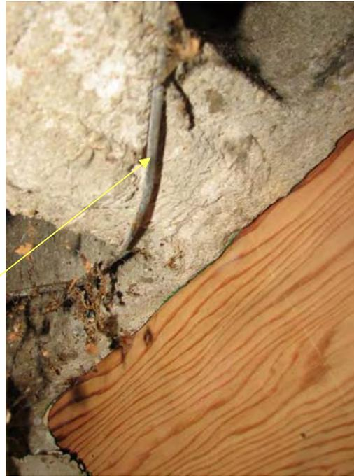
Lots of outside air enters through this hole in the hollow concrete wall— and lots of heat leaves the same way.
