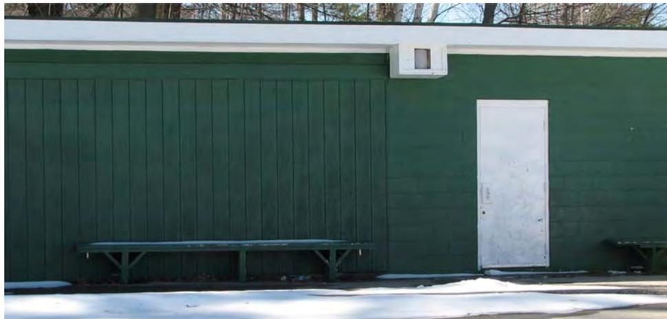
Two sides of the wall have draining capacity, while pavement comes right up to the slab edge on two sides. Best practice would involve breaking up the pavement about 2 feet from the building and installing a perimeter drain near the footing and washed stone. Importantly, it would also allow installing a moisture barrier and insulation at the edge of the slab down to footing if possible. The Tuff N Dri and Warm N Dri system is recommended. A slight paved ramp can be reinstalled at the doors.
