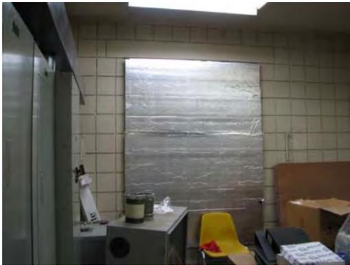
These foam panels were a good choice for covering the large vents previously needed for a generator in this room. However, without being sealed in place, a huge amount of heat is lost (gained).
