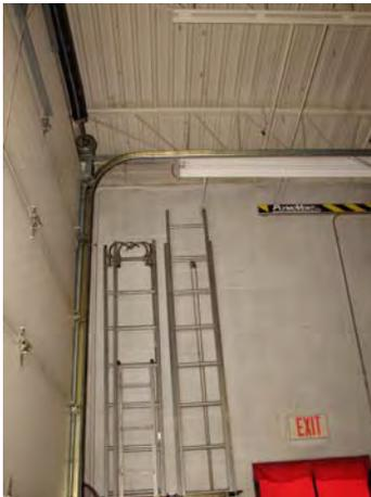
Site visit notes indicate was told that there was 2" rigid applied to outside block wall, but IR suggests otherwise – ie un insulated block walls except where 2x4 insulated cavities exist behind sheetrock.
