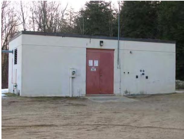
Approx 15' x 33' 12" concrete block on slab with two separate rooms; 10' 2" ceilings under a 10" concrete slab roof. Double metal doors showing signs of vandal attempts.
