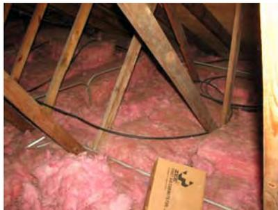
It is always best if soffit vents can be maintained, but equally best if at least 2-3” of foam can cover top plates – and help form an air seal between propa vents and insulation layers. Adequately venting a roof, while effectively air sealing and insulating the ceiling, or attic, is a best practice.
