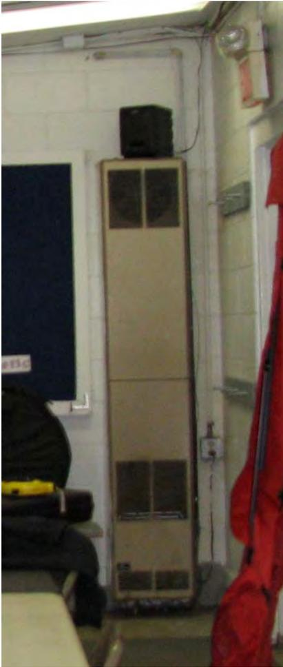
Electric heater mounted near ceiling in the rec or 'computer room'. This room is used after school but less frequently than the rink's warming and concession areas.
