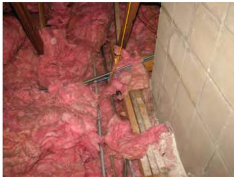
Chimneys can be effectively flashed with metal and caulked with a fire stop; eliminating warm air rising and allowing insulation to be safely installed.
