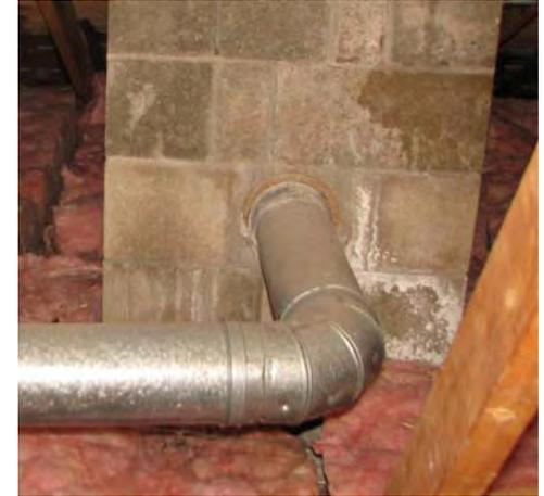
Water leaks around the chimney appear to have been resolved. Smaller leaks may be attributed to either bulk water or repeated condensation pooling near holes in the plastic above the ceiling.
