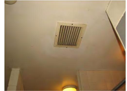
Bathroom exhaust appears to be vented into the attic. Needs to be ducted to outside.
