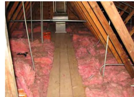
continuous barrier against moisture, air, and heat transfer. Best practice would be to then blow an even 15" of cellulose, but a case could be made to reuse all this material - carefully re-installing these fiberglass batts to a depth of 15" for as many sf as it will cover – then use cellulose for the remainder of the attics.
