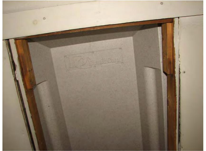
Draft cap helps, but lacking gasket seal.
