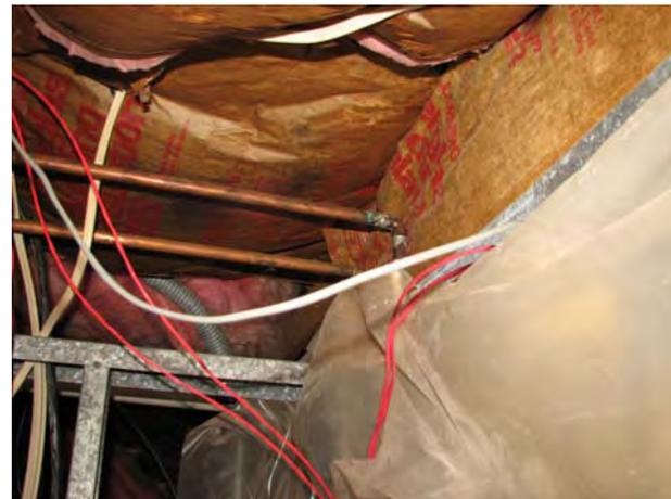
Establishing an air barrier above this ceiling chase will not only reduce heat loss but air transported vapor which, when comes into contact with cold metal or other surfaces, can condense and eventually cause a range of moisture related issues.
