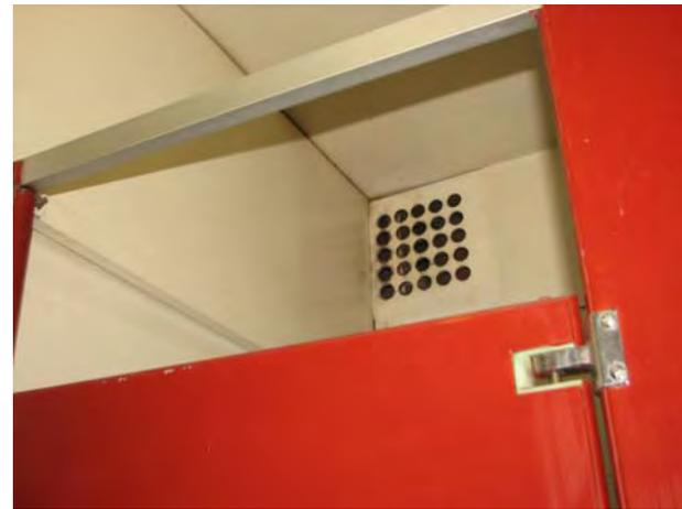
Top corner of bathroom door shows dirt collection as air is pulled from office through bath exhaust.
