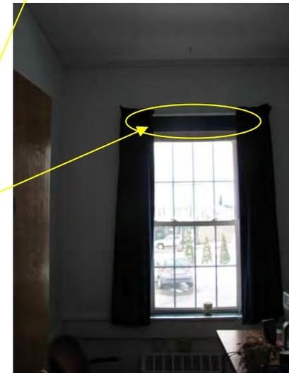
Note that replacement sashes would not necessarily even address this area above which is within the rough opening, but above the window unit. Installation, and details, matter.
