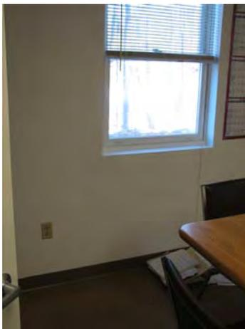
The only two windows are wood double pane with an estimated R value of 2.1. With the lites in the doors, glazing represents approximately 30 sf and just over 1% of wall surface area. Air leaks in at the corners and behind the trim through the rough opening. An effective caulk and weatherstripping would be a cost effective approach to improving these two windows.
