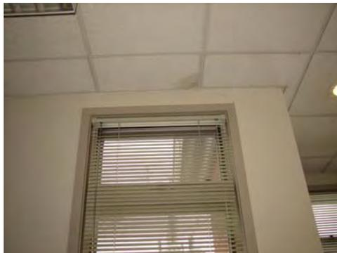
This air leakage is coming from both the attic and the rough window opening. Note the coldest part of the pattern to determine direction.
