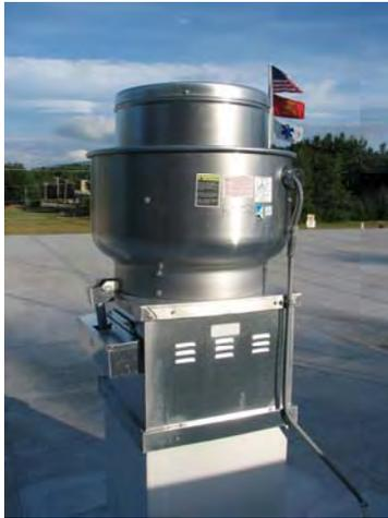
Code compliant stove hood exhaust installed in 2009 per Turner Report recommendation
