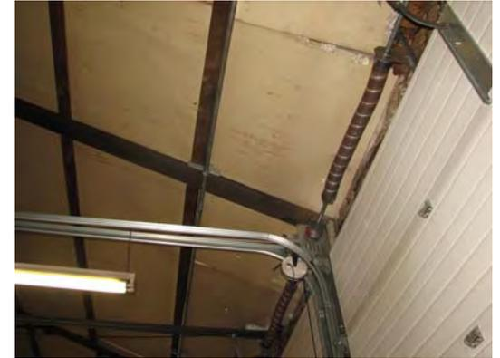
Doors are in fair to good condition and may have an effective value of R6, though large gaps at top, bottom, and sides have a significant impact.
