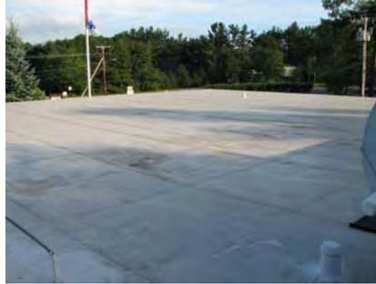
Both roof sections were resurfaced in 1999 by Johnson & Sons. It's considered a 20-year roof membrane, though 4 years left on the warranty.
