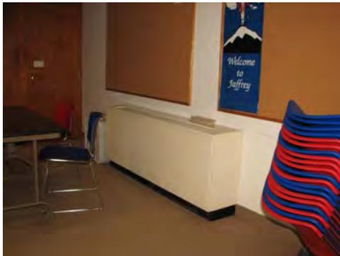
Suspect this would be connected to outside fresh air supply for ventilation requirements in this meeting room, but no evidence of duct work in 2x4 interior wall. And it is known to get 'very stuffy'.
