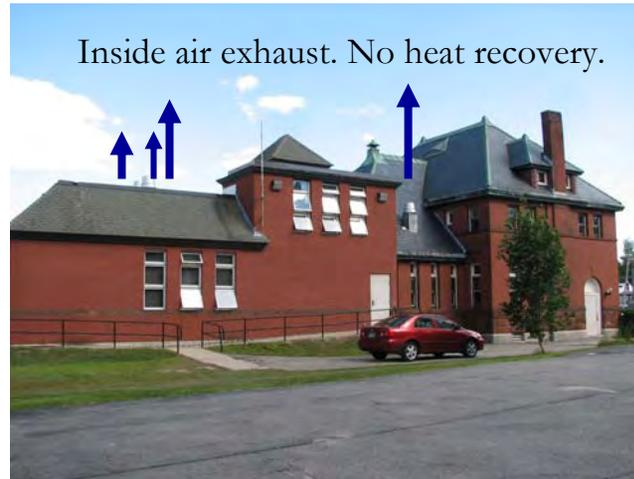
Plus uncontrolled air infiltration and exfiltration, mostly through window and door openings.
