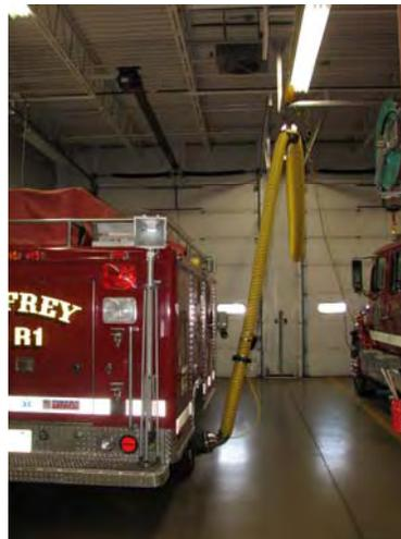
Auto release tail pipe exhaust system great improvement. Still, hot engines also emit a variety of chemically filled fumes and petroleum particles. Building also can have high levels of moisture which is not exhausted through this system.
