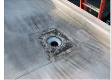
Neither roof drain has screen or leaf trap which increases risk of leaks near the drain
