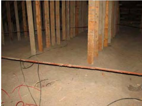
Windows and doors are big, obvious, holes in the envelope. Dozens of wire holes are less obvious but can add up to make one big hole! And when in the ceiling plane, where warm air rises naturally, every hole matters a lot.
