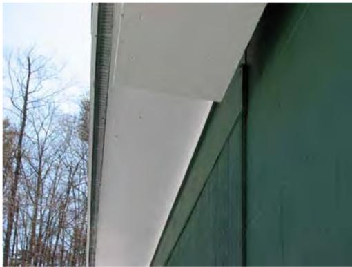
Fairly new standing seam roof may be able to be raised to add continuous rigid. Underneath though any increase in ceiling or roof insulation would likely hold snow longer. Roof is now vented, so soffits would have to be sealed. There appears to be very little room to insulate from inside.
