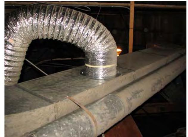
Two inline fans provide exhaust from the basement. As the building is further tightened to reduce heat loss, this continuously running exhaust fan could depressurize the basement enough to cause back drafting in the boiler room.
