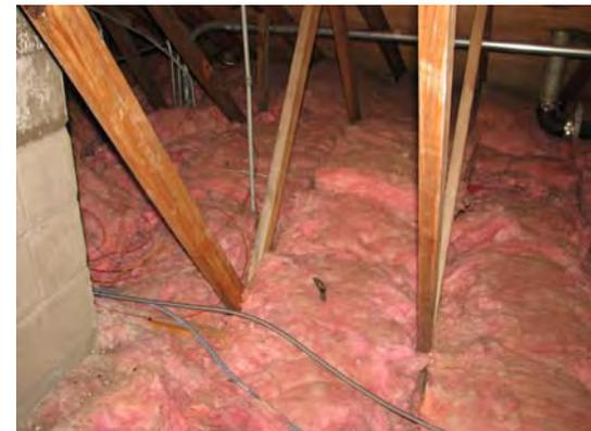
Conventional ‘energy efficiency’ improvements focused on the inexpensive approach of adding more insulation on top. Without comprehensive air sealing, and careful installation of effective insulation, these well intended efforts can make a relatively minimal difference. Unfortunately, meaningful improvements are more labor intensive – particularly when there are past efforts to work around. Fiberglass is rarely the optimal insulation for NH’s climate.
