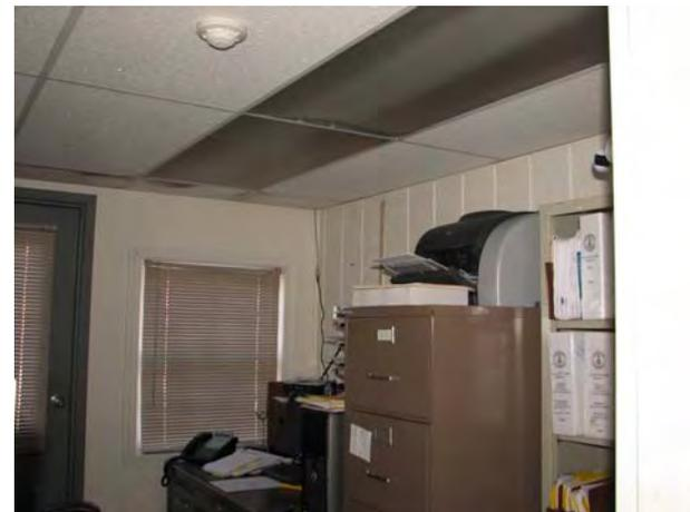
Water damage from past leakage
