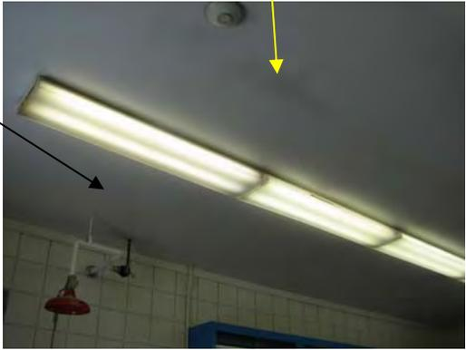
Its not a coincidence that the stain on the ceiling aligns with coolth pattern. Thermal bridging – conductive material in contact with both inside and outside surface – can cause condensation on interior spaces as warm moist air contacts with a surface below the dew point.
