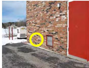
The louvered vent to the left appears to be the former strategy to introduce combustion make up air but is no longer used so is now just a hole in the envelope.
