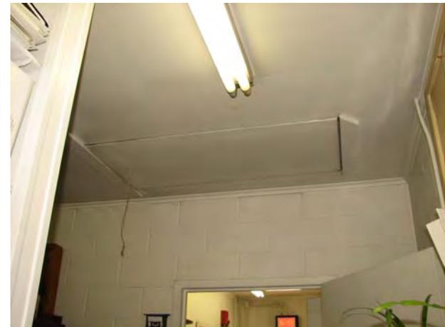
Even after insulation had been added, without an air barrier or continuity, there is still significant heat loss into the attic.
