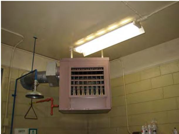
Reznor Propane heater with electric fan. Set to 70°F year round with low temp alarm.
