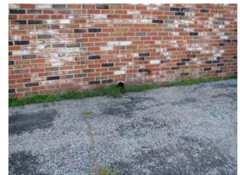
Mold and dirt accumulate near cracks and gaps where exfiltration takes place.
