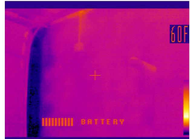
Doors are in good condition but still allow air leakage along the tracks.
