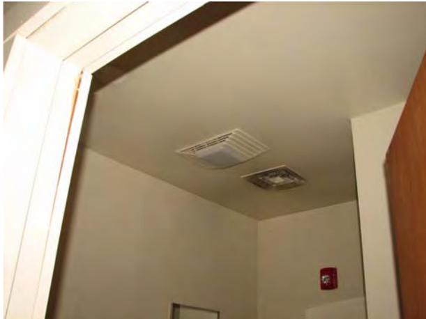
Pressure diagnostics indicate a fair amount of air leakage from the ducts in the chase, most likely at the seams and where the ducts connect to the registers. Again, an air barrier and effective insulation above will more effectively bring these ducts into conditioned space, thereby reducing energy loss. However, sealing all seams and junctions would reduce heat loss further by directing heat below the drop ceiling more efficiently.
