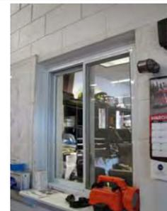
The wall between a garage space and 'living' space is an important air barrier to maintain for moisture and air quality. Since the bays are a separate heating zone and often kept cooler, it is also an important heat loss barrier as well.
