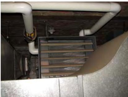
Converting to a sealed combustion boiler will allow sealing of combustion make up air fan and eliminating this mechanical room space heater.
