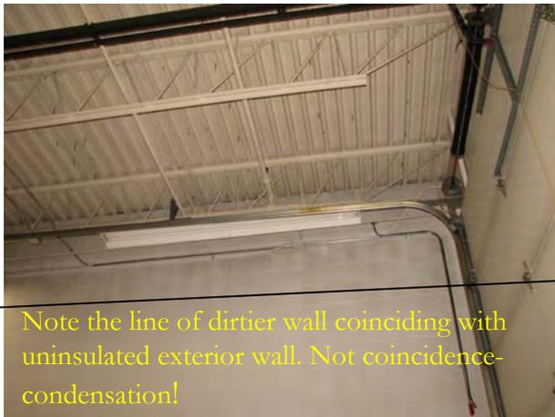
Note the line of dirtier wall coinciding with uninsulated exterior wall. Not coincidence-condensation!
