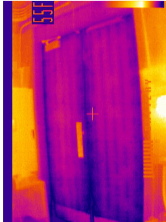
Significant heat loss through un insulated doors, slab, and walls and suspected minimal roof insulation.
