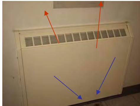
No fan, kitchen room with passive convective looping from radiated heat
