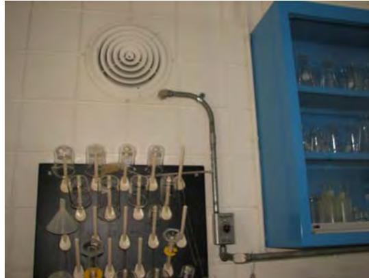
Manually operated timed wall exhaust in lab.
