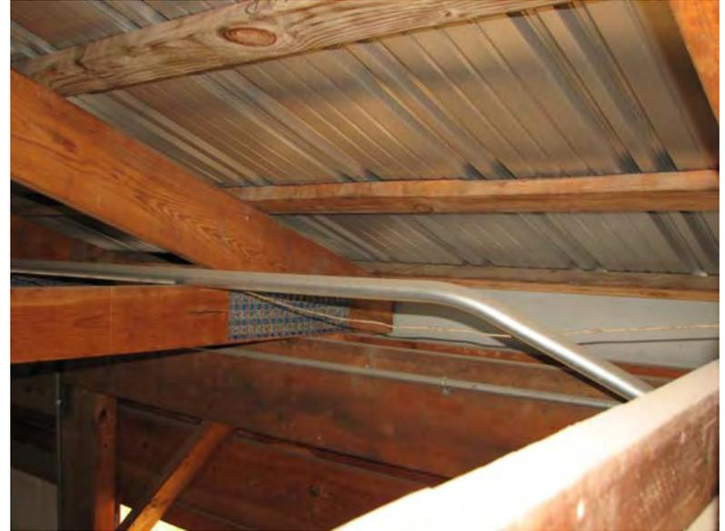
Insulation strategies would involve detailing a continuous air barrier in direct contact with a continuous insulation barrier on the walls and connecting with the ceiling – while still providing for a vented roof.
