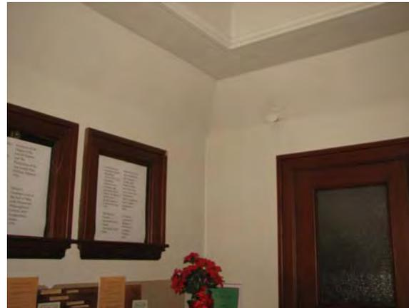
This connection between conditioned and unconditioned space is significant – especially and partly because of the high temperature of this corner on the 2<sup>nd</sup> floor. The attic should not be 60° - a result of an inadequate air and thermal barrier; but this room corner should not be heated to 80°. That's an issue of the heating and distribution system.
