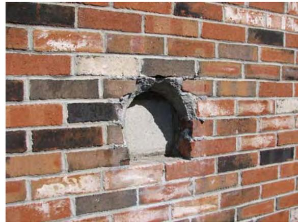
This hole, now sealed, indicates a minimal air space, if any, behind the brick veneer. Is it vented at top or bottom? Exterior insulation strategies would be effected by the answer..
