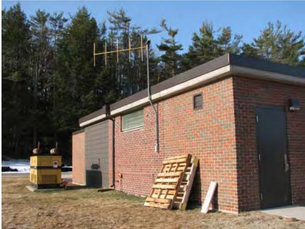
Approx 22' x 34' (12") concrete block with brick façade over 9' ceilings under 10" concrete slab roof 748 ft<sup>2</sup> and 6800 ft<sup>3</sup>; 1812 ft<sup>2</sup> surface area of shell. Three distinct rooms with separate heating and ventilation and a covered port out back.
