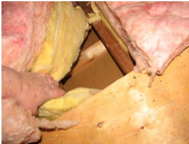
The challenge here is that there is no solid floor or ceiling below. While it would have been relatively inexpensive to create during initial construction, it is considerably more expensive to install after the fact which can make the cost/benefit analysis fall outside conventional energy efficiency formulas. Even so, establishing a continuous air barrier at this ceiling plane is the number one recommendation..
