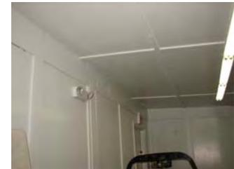
The framed section of the building appears to have more thermal bridging, suggesting bats only – in between 6” rafters would indicate approximate R15-16. Snow on this section confirms it may be slightly better insulated than the first room – but also that this room is generally kept at a lower temperature.
