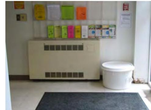
Entry fan coil unit - Forced warm air only, not connected outside fresh air
