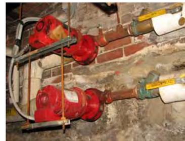
By converting the heat coils, variable speed circulating pumps would also improve efficiency.
