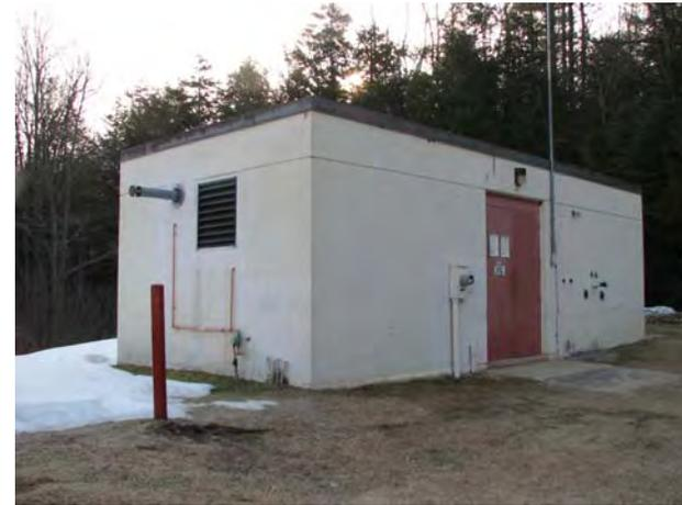
Uninsulated and well vented building uses between 650-900 gallons propane a year for heating and emergency generator. Impossible to know how much of the fuel is used for the generator.
