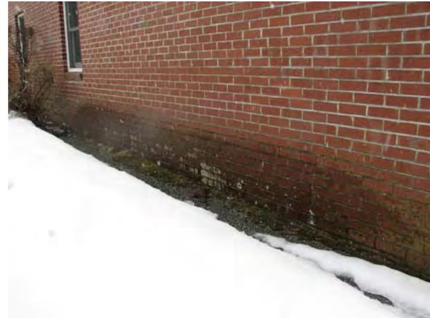
Insulation gaps in envelope create greater conductive heat losses.
