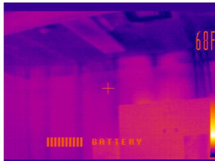
Establishing an air barrier above this dropped ceiling in direct contact with effective insulation levels will make a dramatic improvement in comfort and reduction of oil use.
