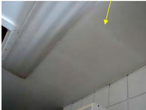
Faint, but here you can see the same situation in reverse! Where the ceiling is warmest where the 1.5" wood joist is touching the ceiling. Cavities here are sparsely, or not at all, insulated.
