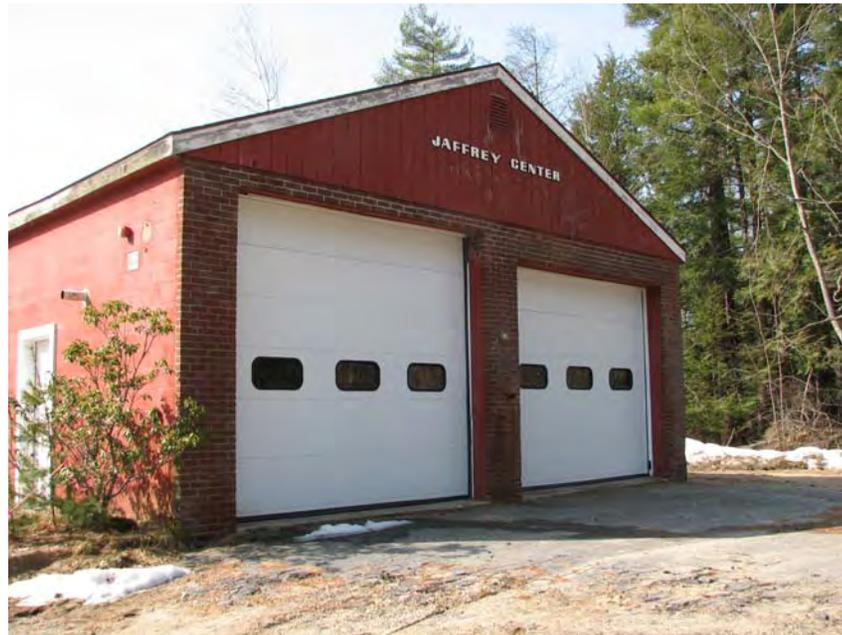
Rectangular, 2160 ft<sup>2</sup> (30 x 72) uninsulated concrete block, brick façade on north side with two overhead doors, and “cold” roof.
