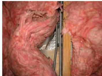
2x6 joists with 6" fg batts over layer of poly with holes and a layer of Reflectix. Then a 9" chase above dropped ceiling tiles. No continuous air barrier.
