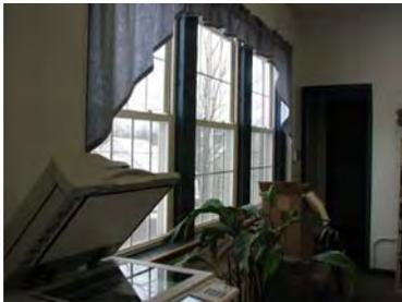
In spite of what was written on an earlier slide, a case can be made to install new windows if the existing ones don't close anymore. Vinyl replacements are notorious for becoming less and less tight over time. Still, the most important thing is to stop air – and that can be done without buying new ones. In addition, new windows don't guarantee tight fits! The rough
