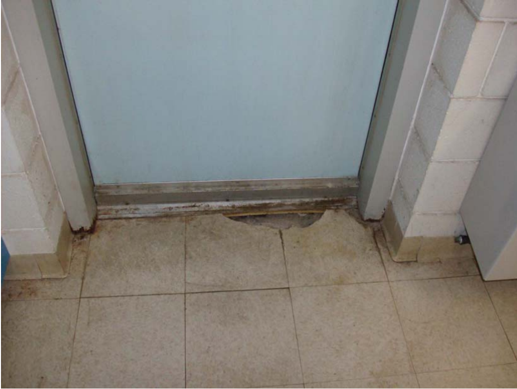
Damaged Tile at Laboratory Door
