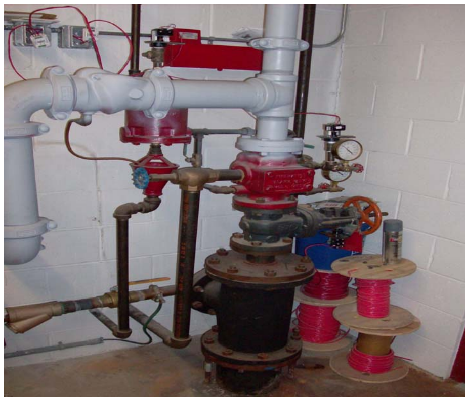
Water Supply Entrance for Domestic and Sprinkler Supplies
