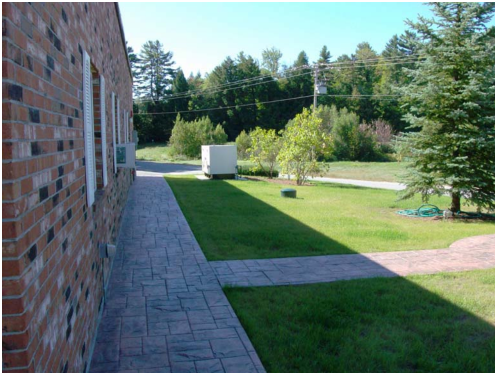
West Side of Station – Note Stamped Concrete Walk and New Gas-Fired Generator
