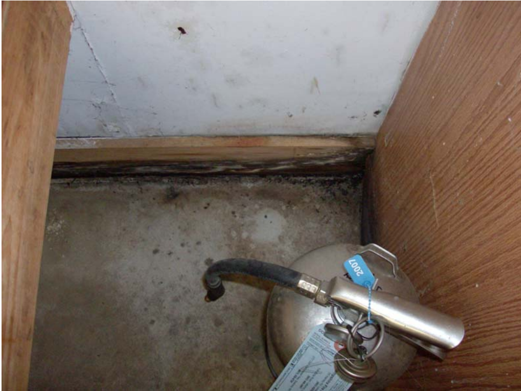
Water Damage and Mold Along Baseboard
