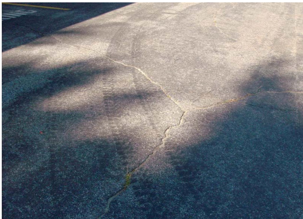
Cracks in Pavement at Front of Station
