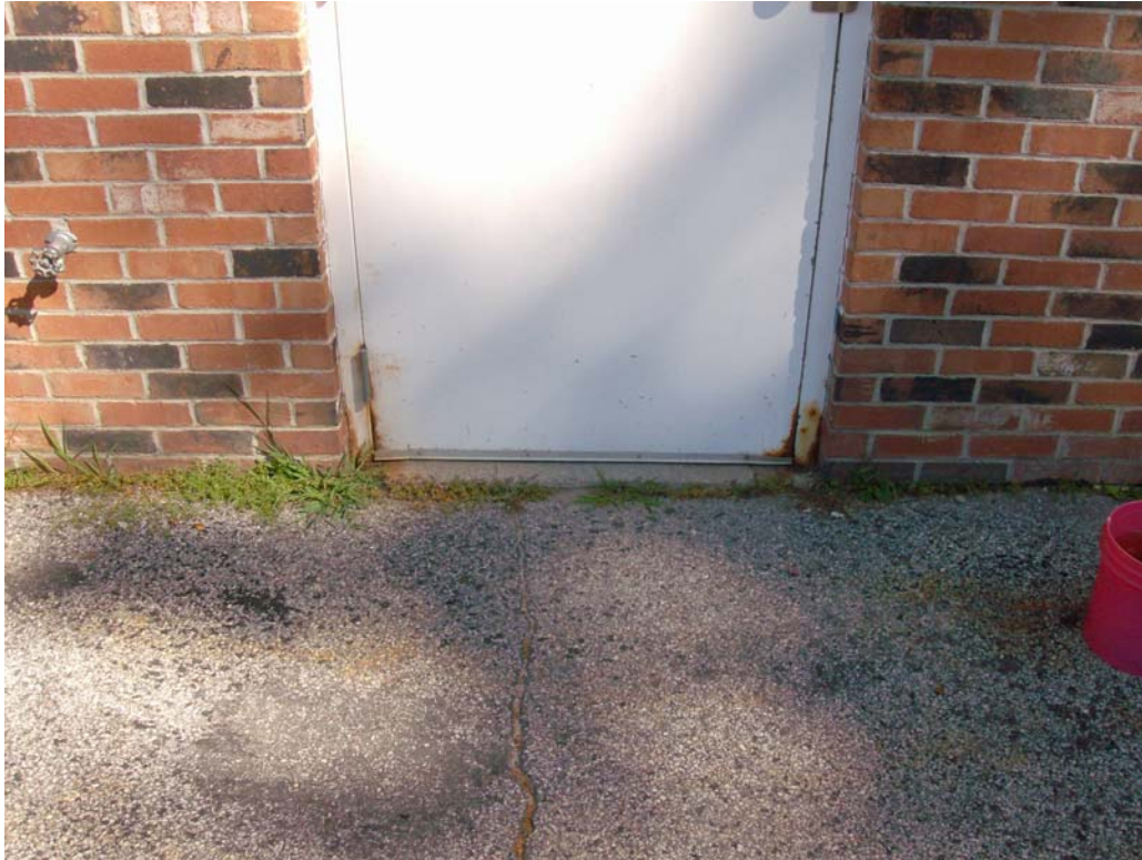
Man Door at Back of Station – Note Rust on Frame and Bottom of Door
