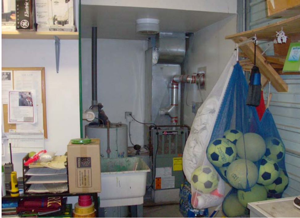
Furnace, Water Heater, and Slop Sink – Garage of Parks and Recreation
