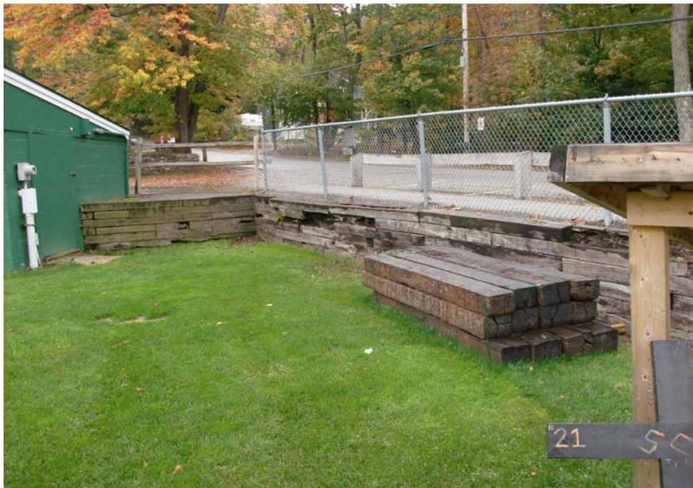
Wood Retaining Wall Along Howard Hill Road
