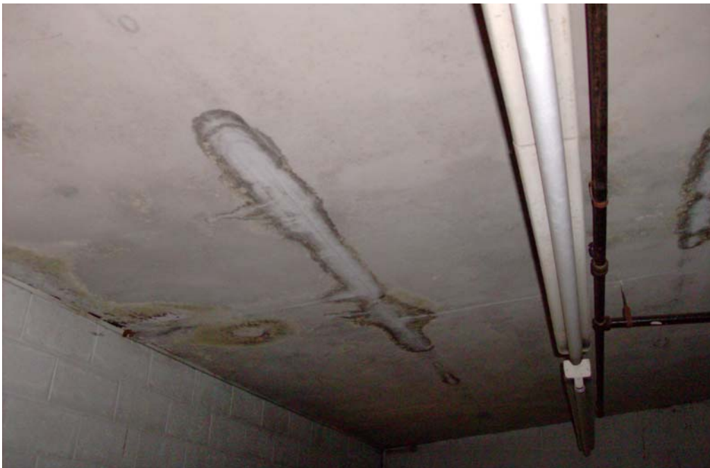
Moisture Intrusion in Storage Area
