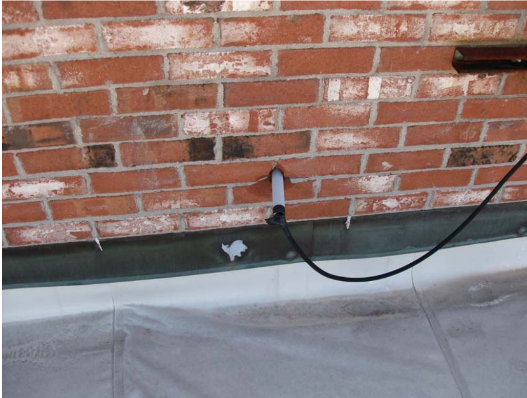
Wall Penetration for Antenna Cable at Roof Parapet
