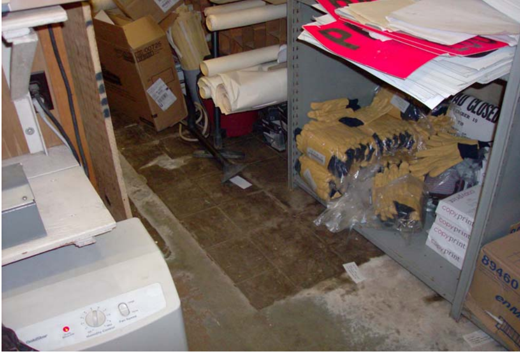
Storage Room – Note Old Asbestos Floor Tiles
