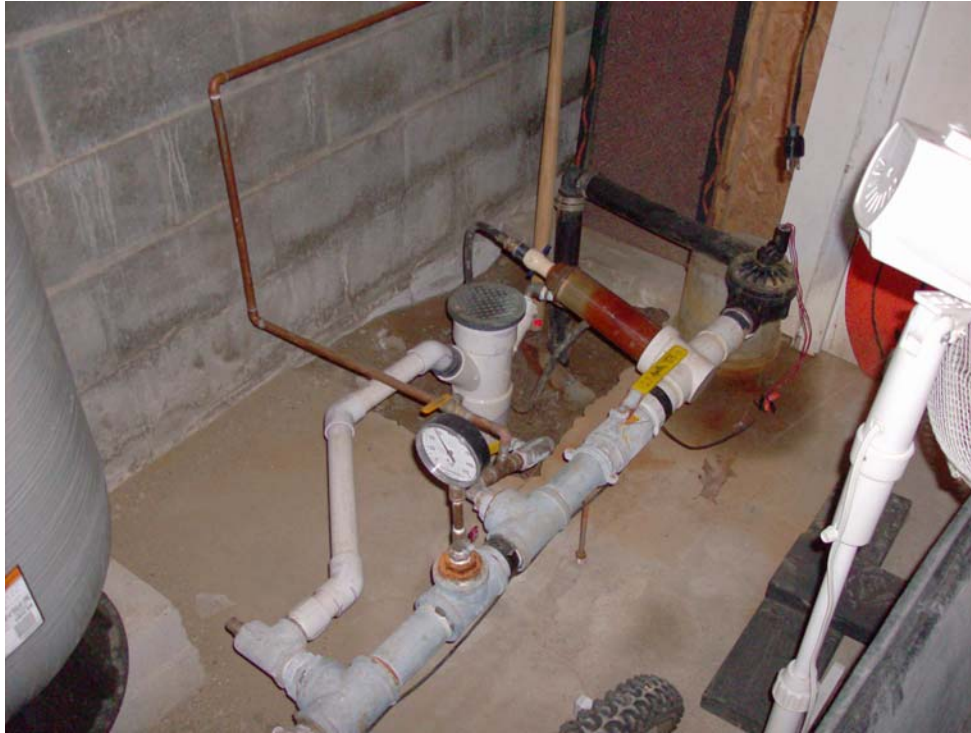
Incoming Water Line from Well for Irrigation System
