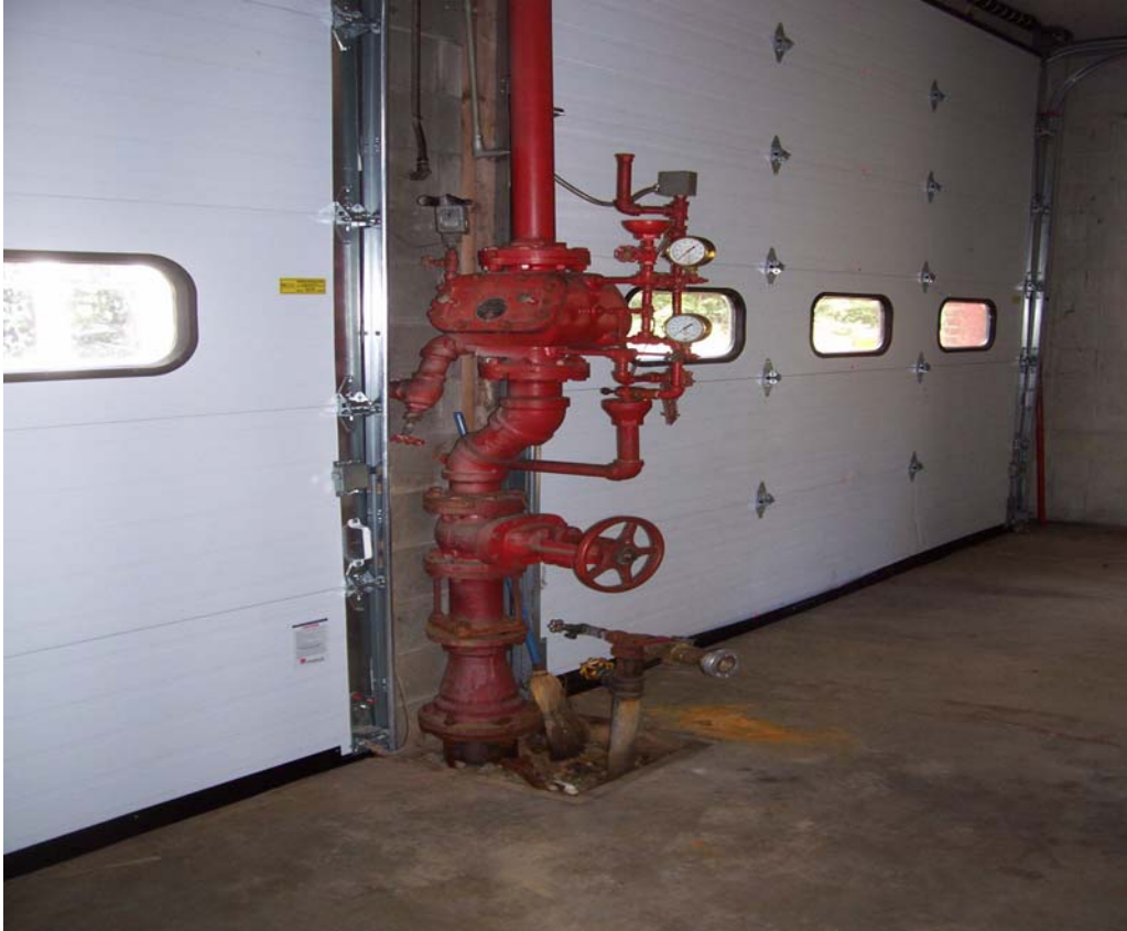
Point of Entry for Sprinkler System
