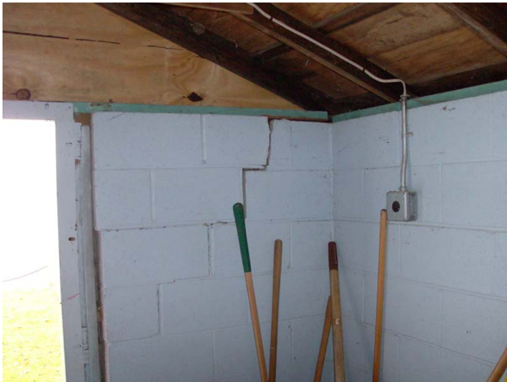
Crack in CMU – South Wall of Changing Room
