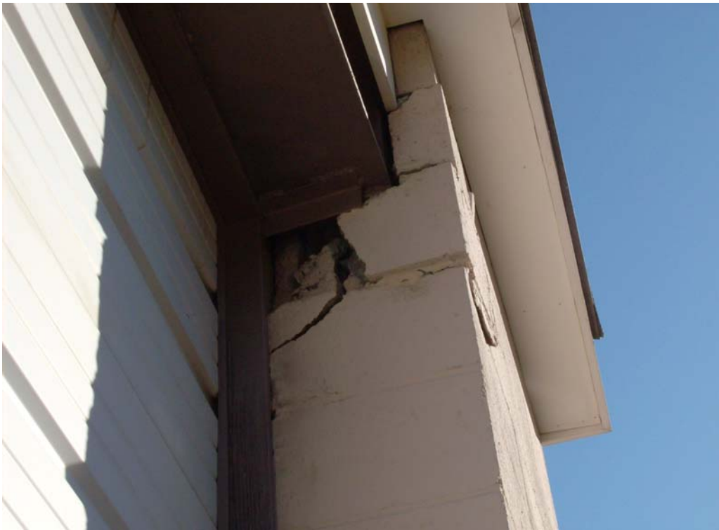
CMU Damage at Overhead Door – Southeast Corner of Garage
