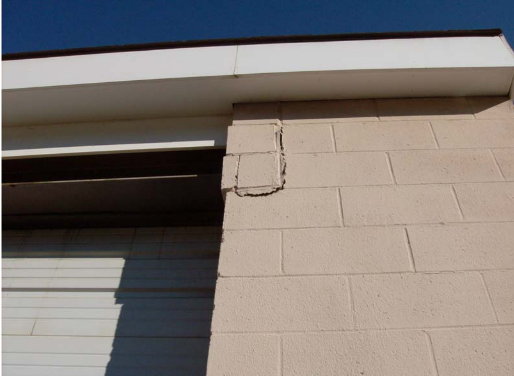
Damage at Head of Overhead Door – Southeast Corner of Garage
