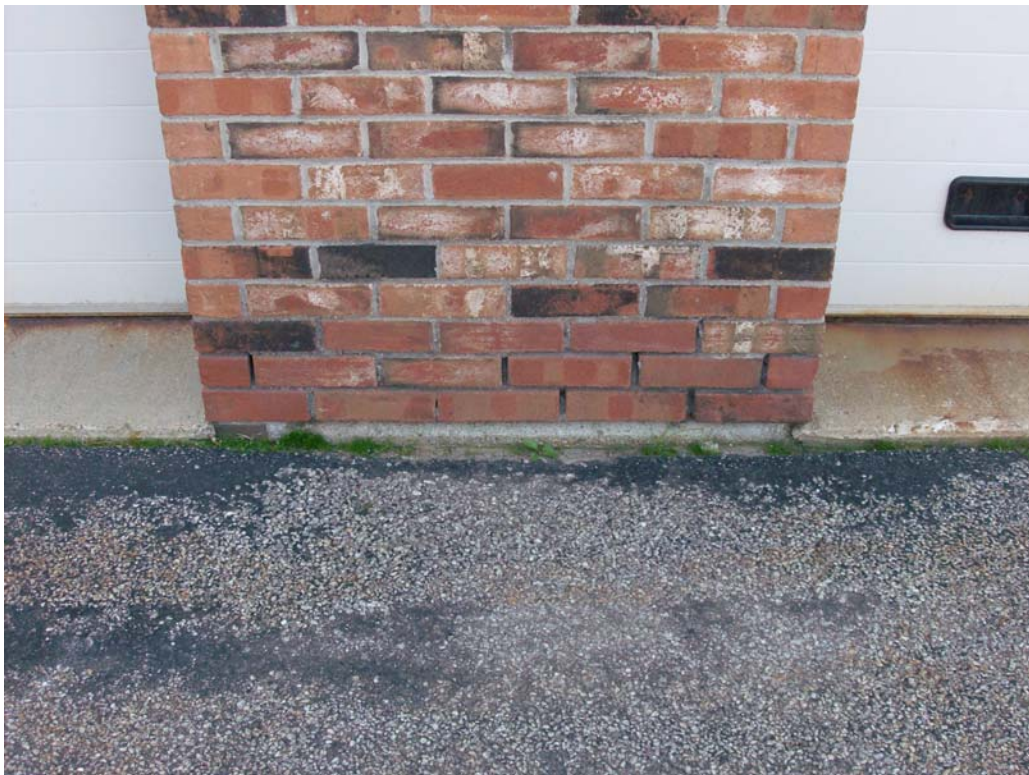
Mortar Loss in Joints at Lower Brick Courses
