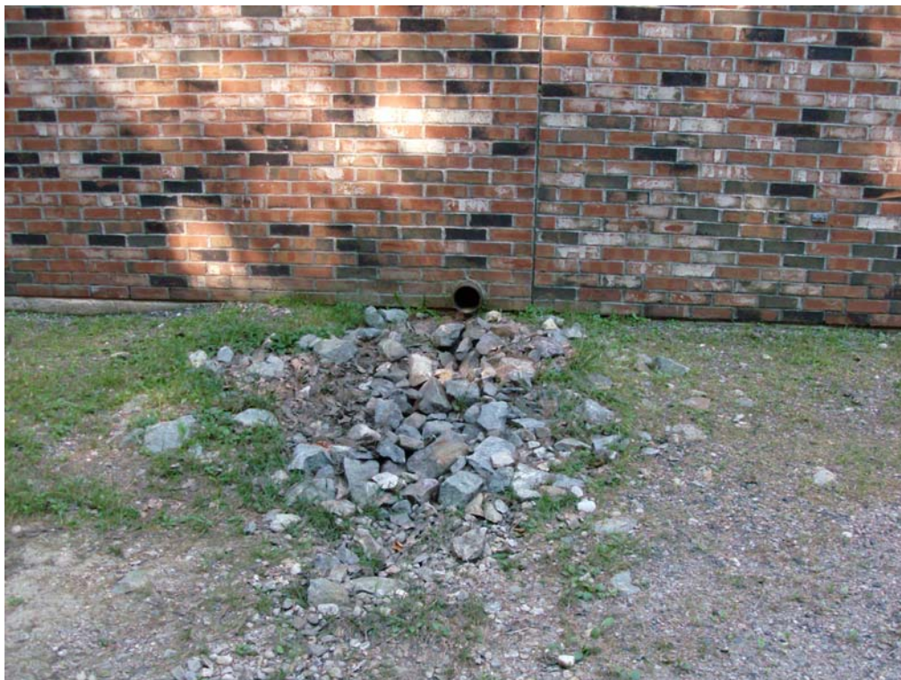
Roof Drain Termination on East Side
