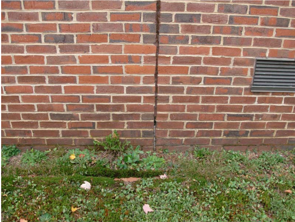
Typical Brick Control Joint
