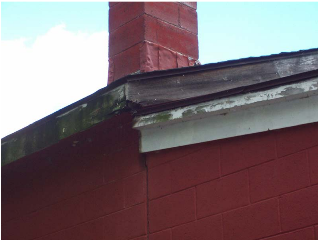
West Side – Note Rotted Trim, Peeling Paint, and Chimney in Need of Re-pointing
