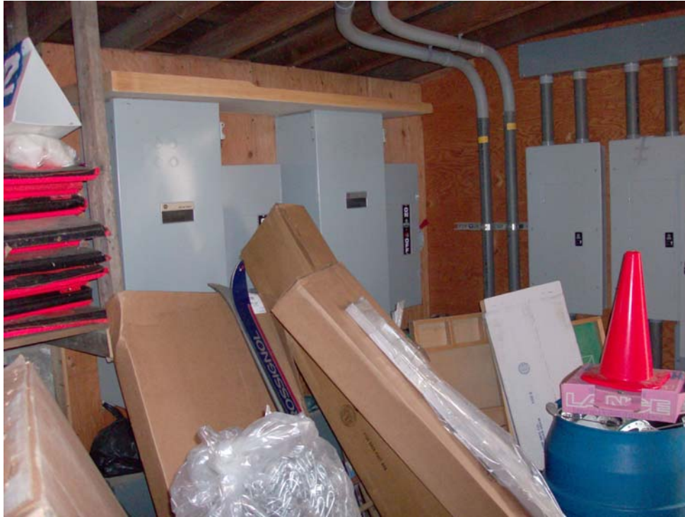
Electrical Panels in the “Dungeon” – Note Boxes and Debris Blocking Panel Access
