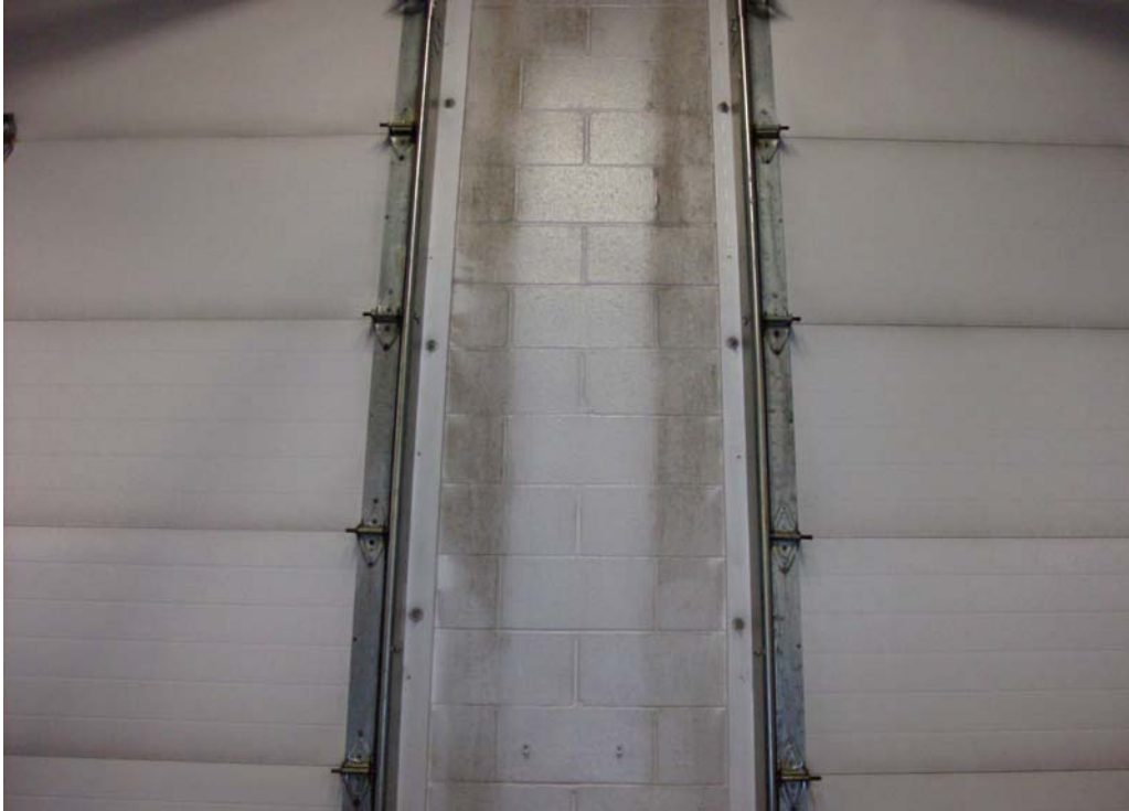
Discoloration on Walls Adjacent to Doors
