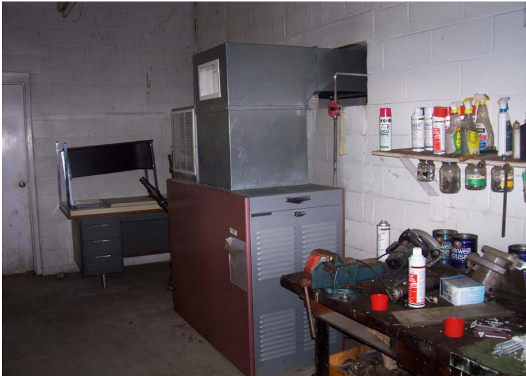
Oil-Fired Hot Air Furnace
