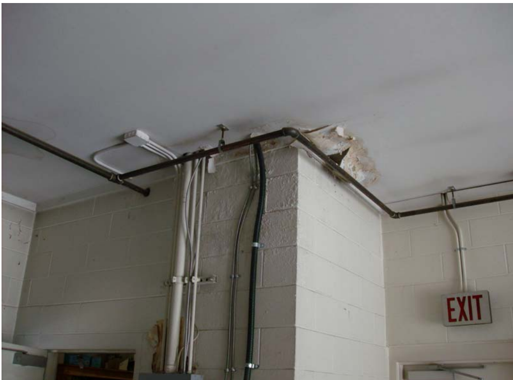
Prior Water Damage Around Chimney in Garage
