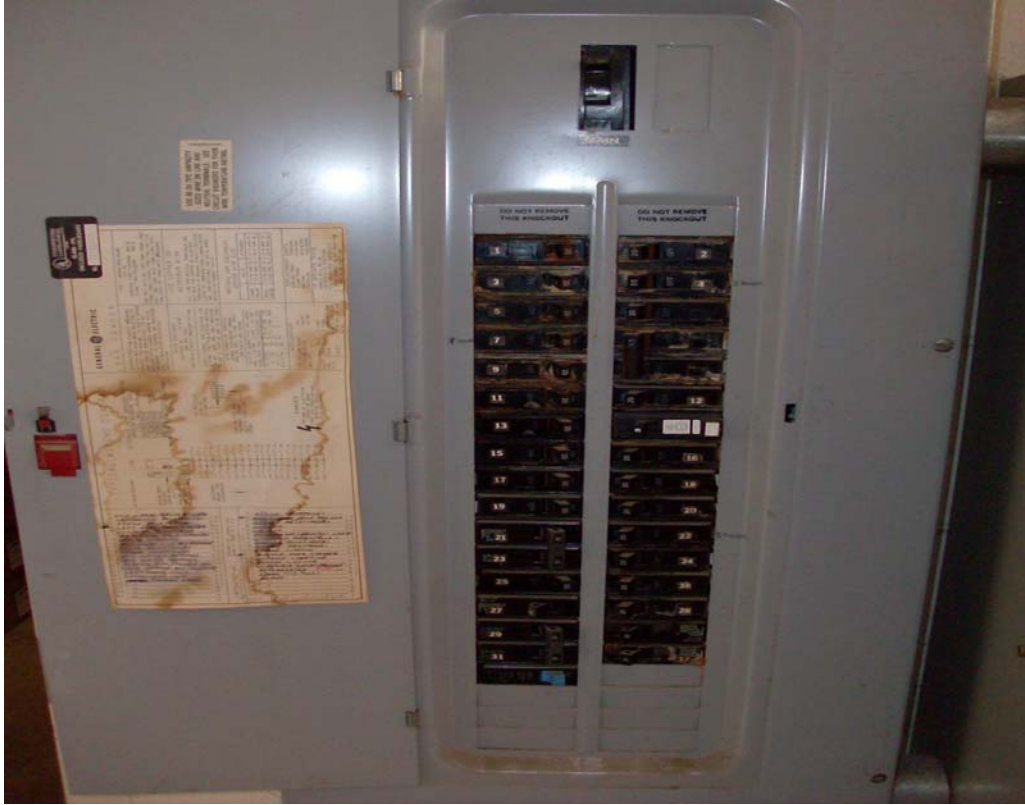
Water Damage in Electrical Panel
