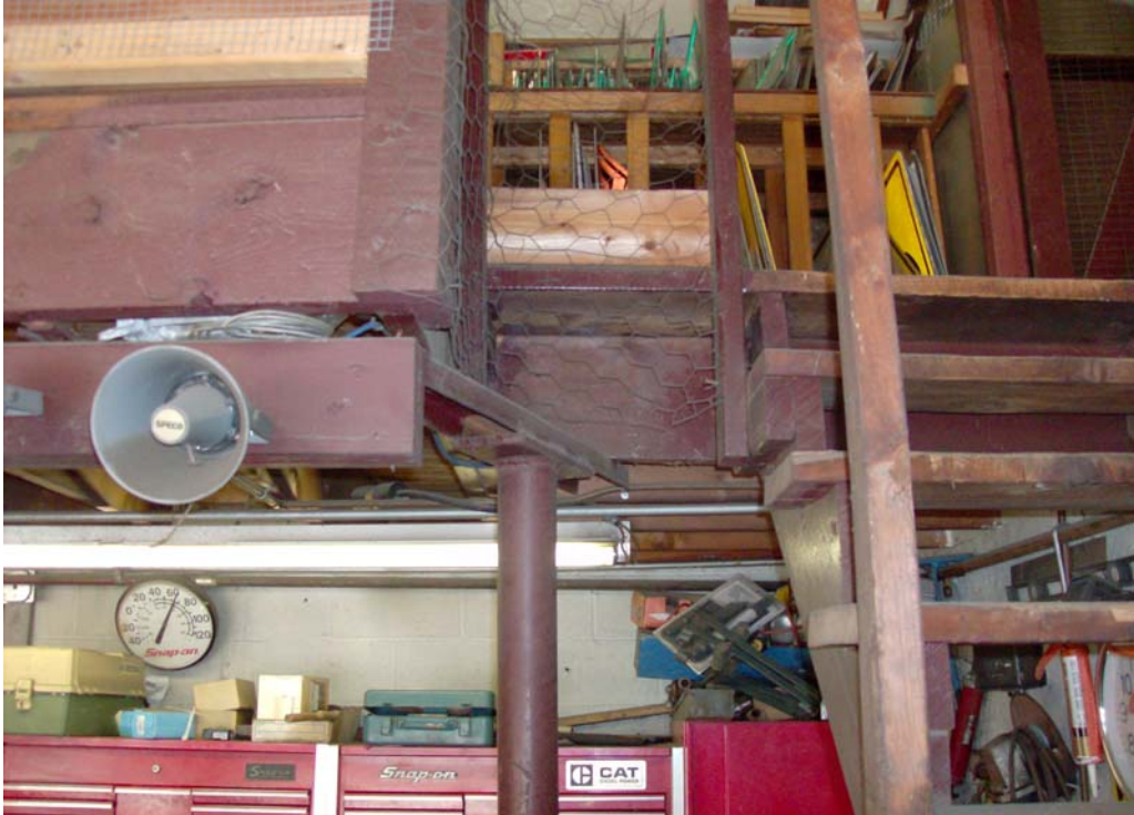
Unconventional Support for Outside Corner of Mezzanine
