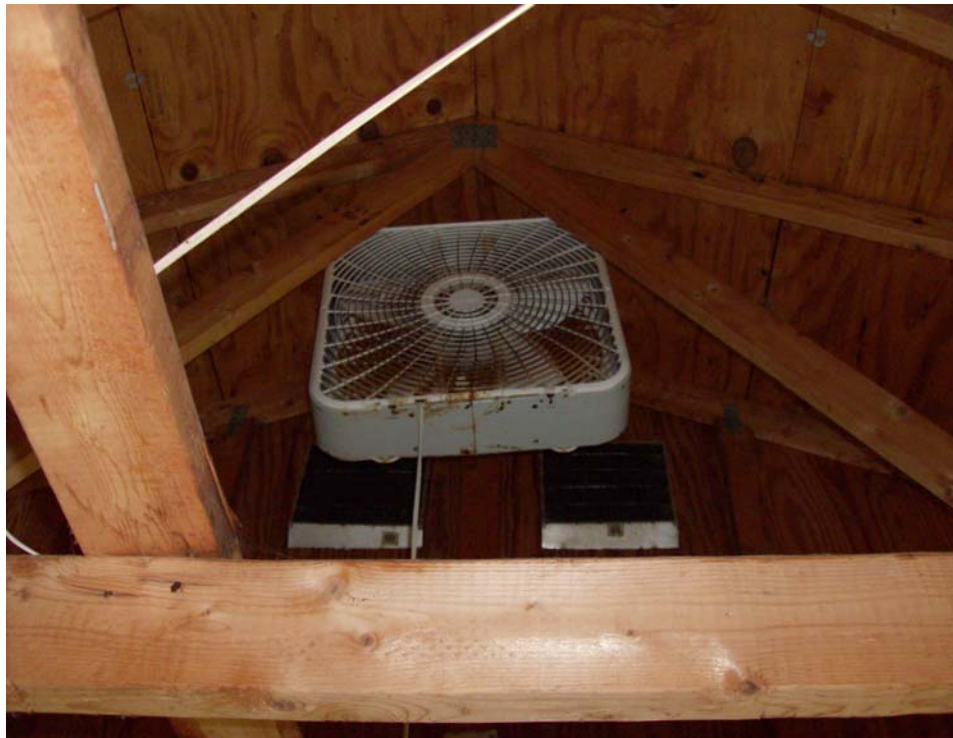
Box Fan Used to Vent Cooking Fumes and Smoke
