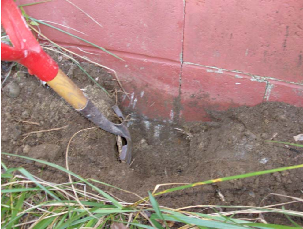
Existing Grade Covering Lower Block Course and Weep Holes
