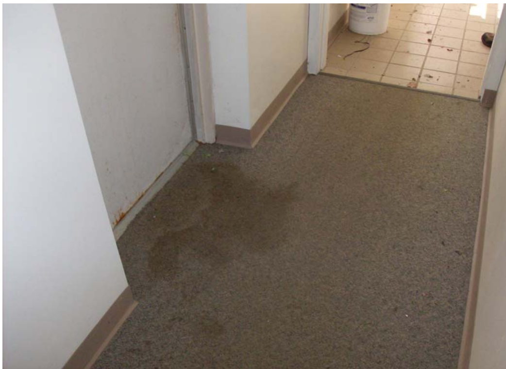
Stained and Water Damaged Carpeting at Rear Entrance
