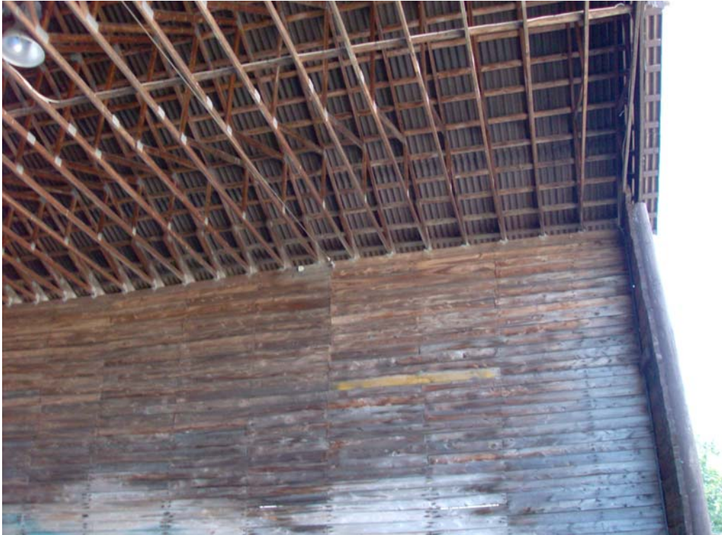
Roof Trusses and Wood Covered Walls in Salt Storage Shed
