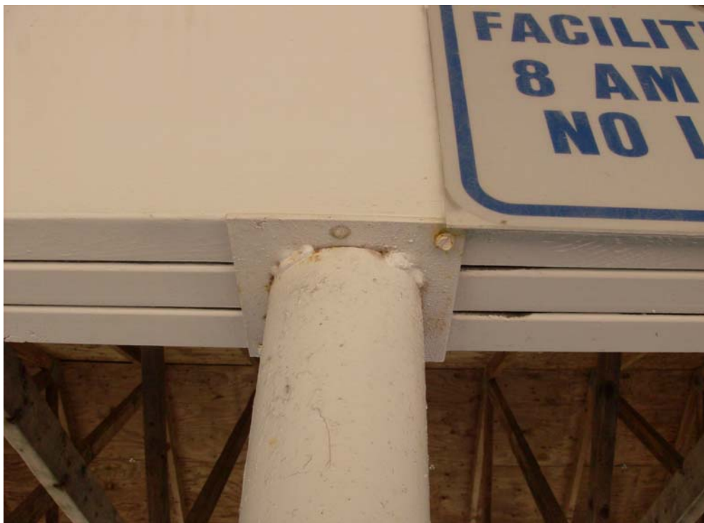
Beam to Column Connection – Roof Over Picnic Area
