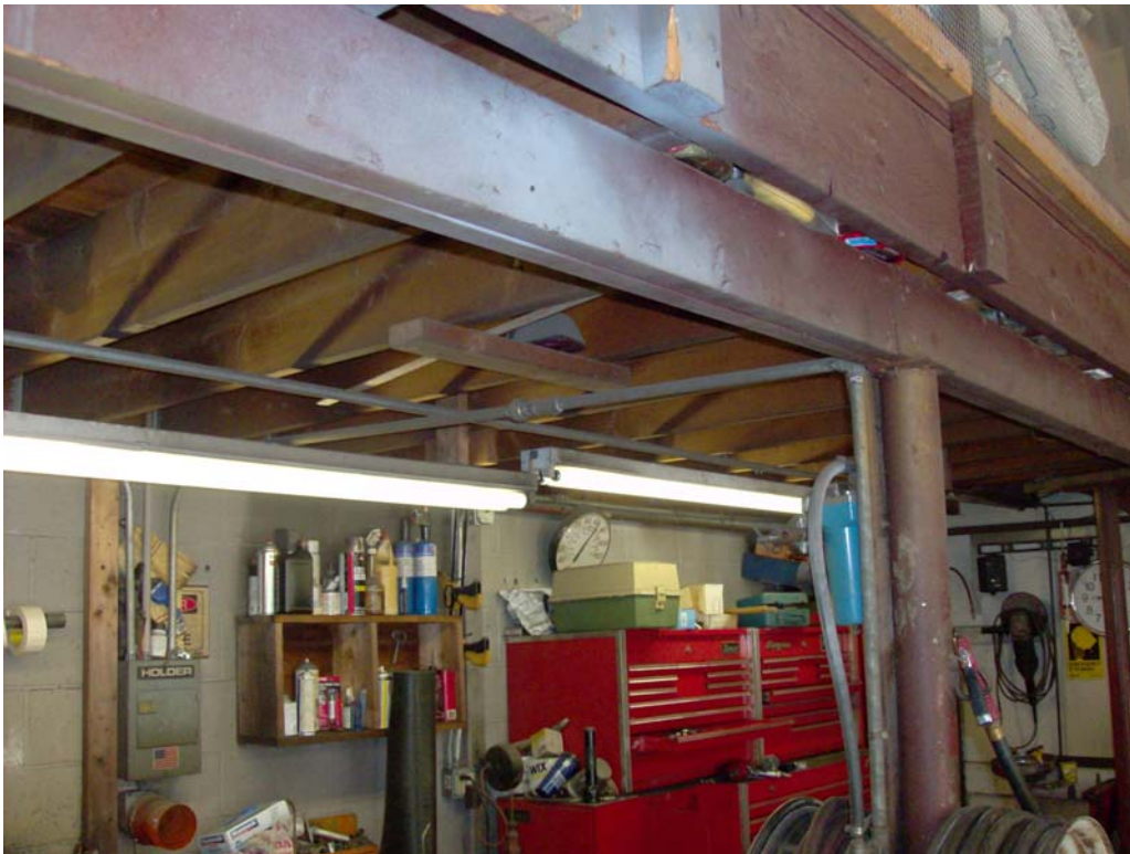
Wood Framed Mezzanine Along North Wall of Garage
