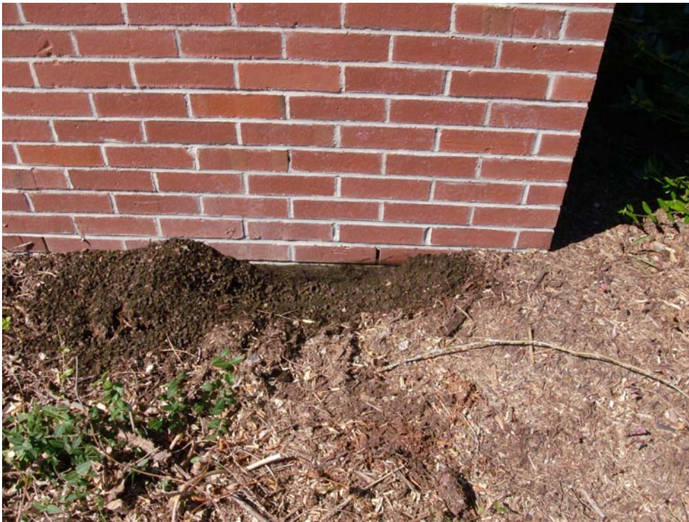
Soil and Mulch Blocking Mortar Joint Weeps
