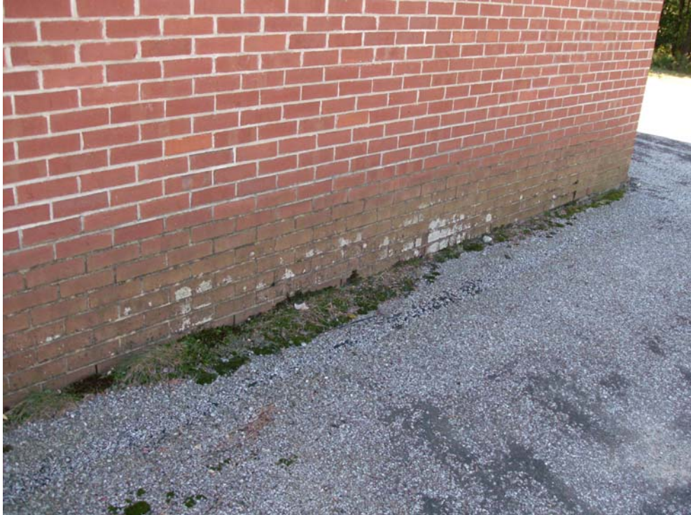
Water Damage and Moss Growth on Northwest Corner
