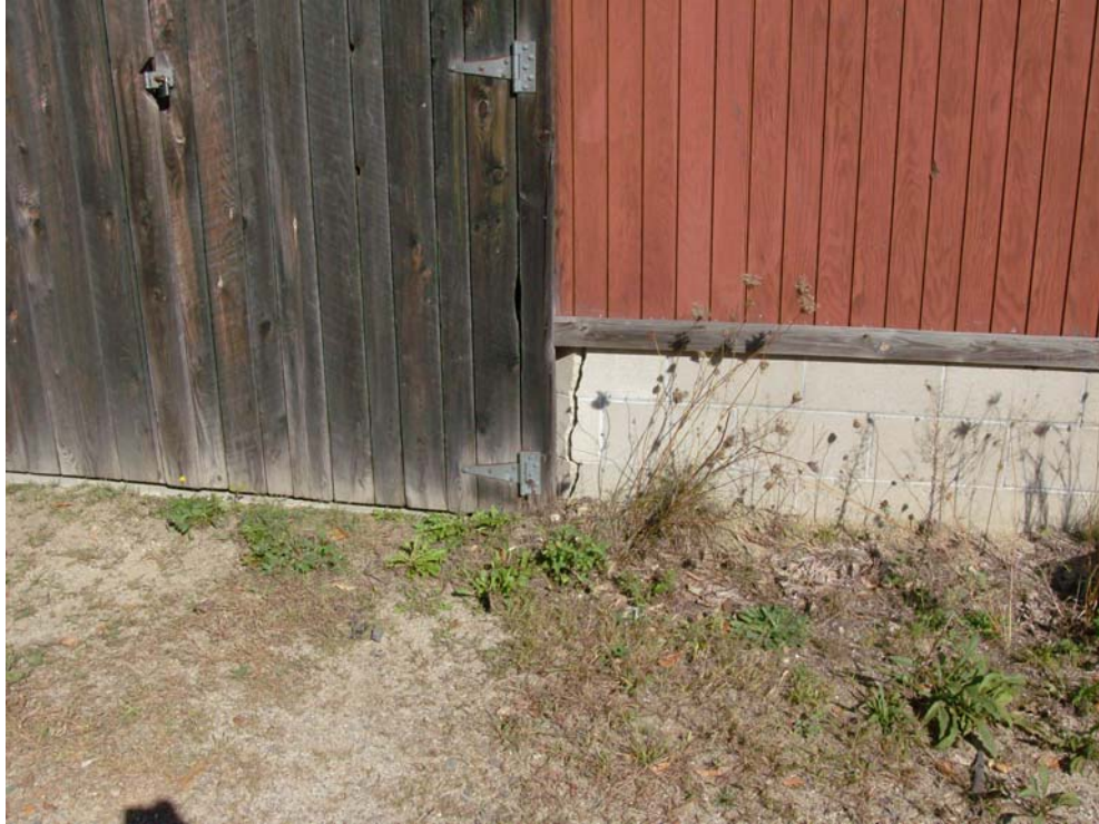
Damage to CMU Foundation of Storage Shed
