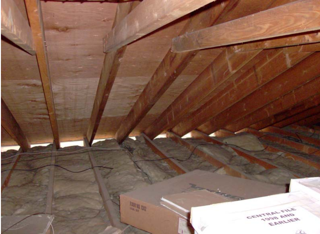
Typical Wood Framing Above Administration Wing – Note Old File Storage
