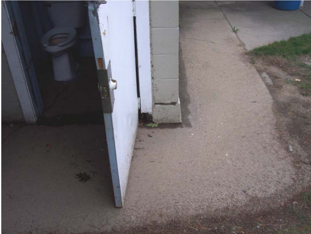
Damaged Door at Bathroom – Rear of Bath House
