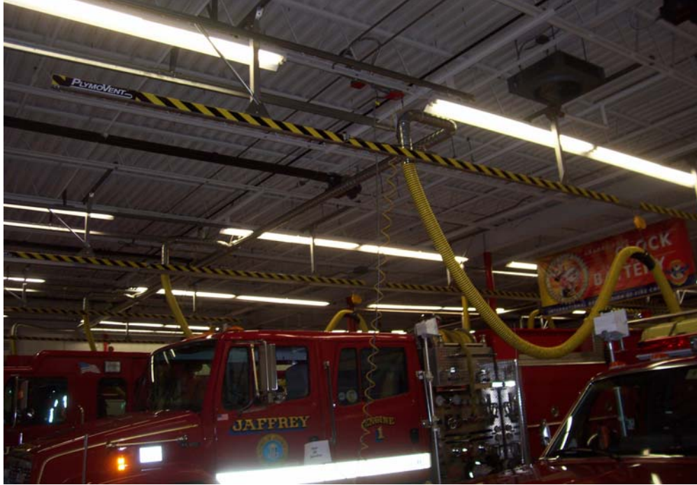
Plymovent System for Exhaust Removal
