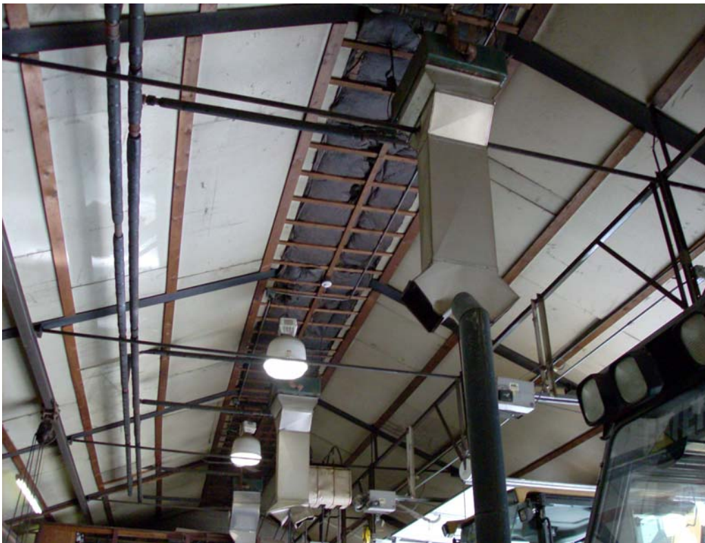
Insulated Roof of Equipment Bays
