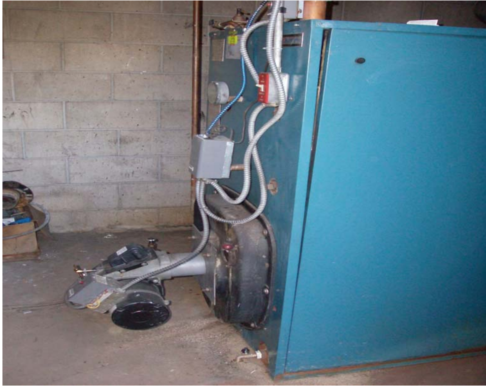
Oil-Fired Hot Water Boiler
