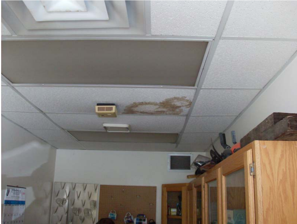
Water Damaged Ceiling Tile in Lab Area
