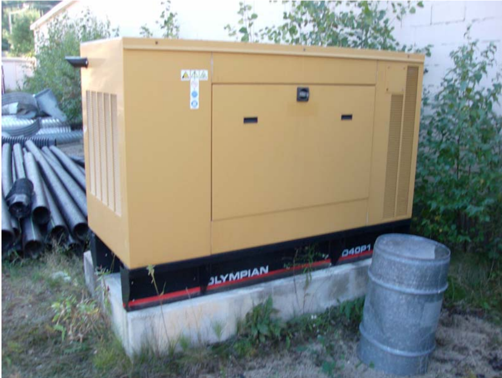
Diesel Oil Fired Emergency Generator at Rear of DPW Garage
