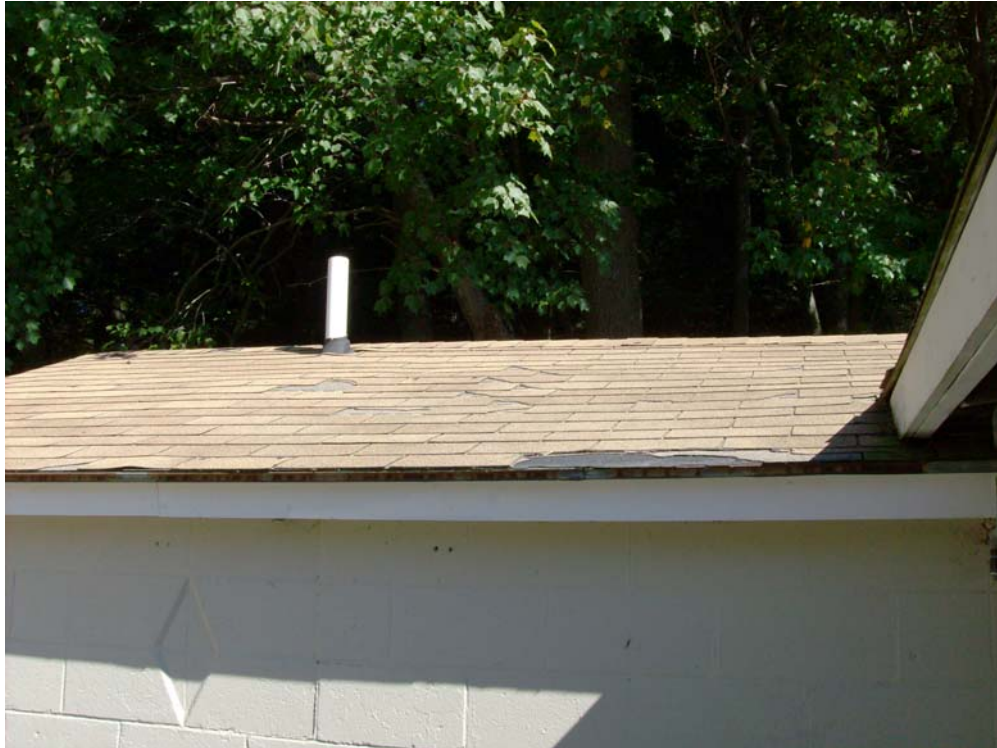
Missing Roof Shingles Over Bath House
