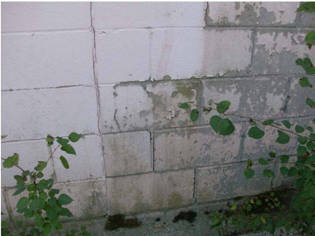
North Wall of Garage – Note Cracking, Peeling Paint, and Moss Growth
