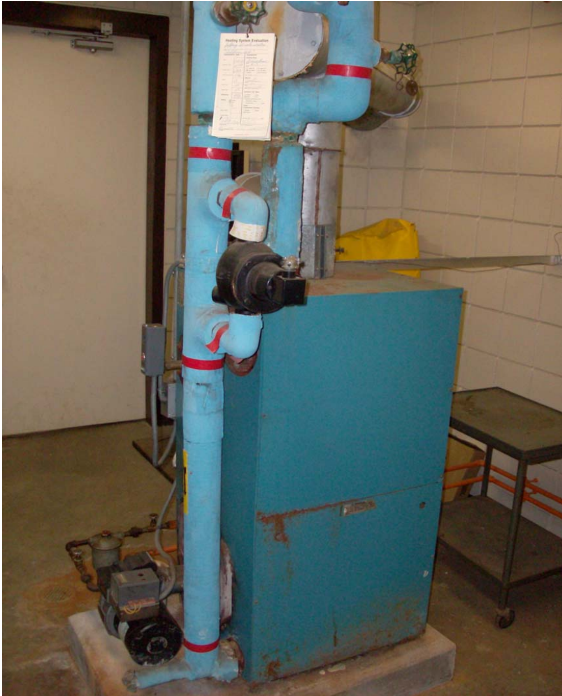
Oil-Fired Boiler for Forced Hot Water Heat
