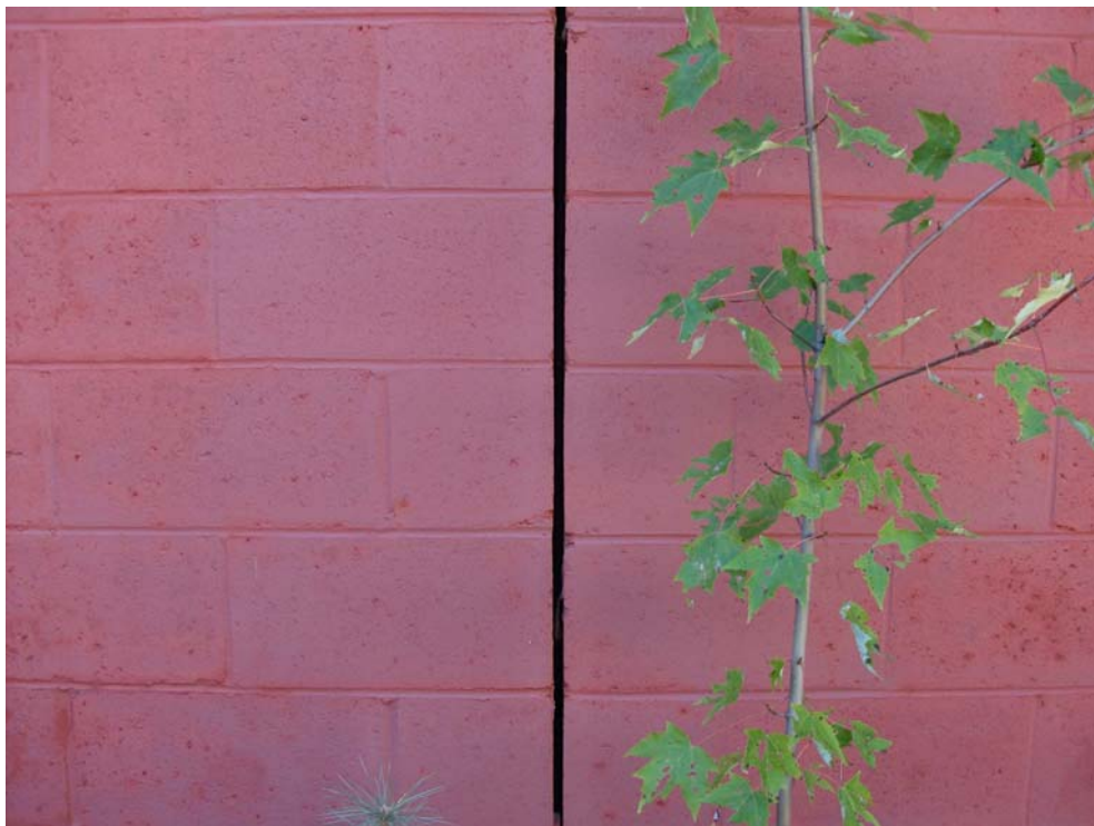
CMU Control Joint in Need of Caulking
