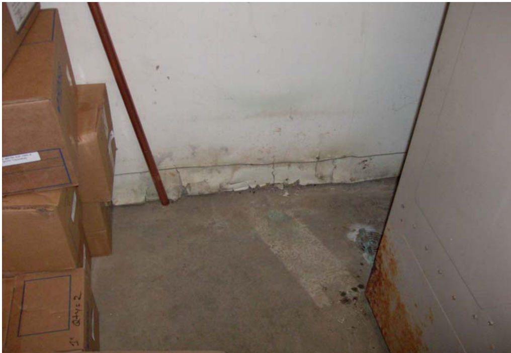
Water Damage Along Wall – May be from Leaking Water Heater
