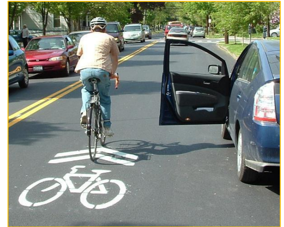
A shared lane marking, or sharrow, placed outside the "door zone" of parked cars. Source: Cycling Action Network.
