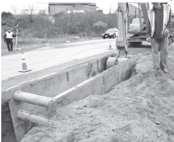
Water main construction underway on Old Sharon Road (Stone Bridge TIFD Project)
