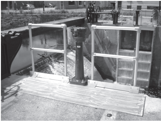
New gates and control mechanisms at Main Street Dam
