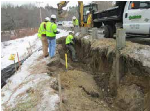
Repairs were made to the sanitary sewer on Peterborough Street in December prior to cure-in-place lining by Insituform as part of the Town's sewer inflow/infiltration program
