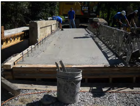
Alternative I Rehabilitation with Cast-in-Place Concrete Deck Replacement over Arch
