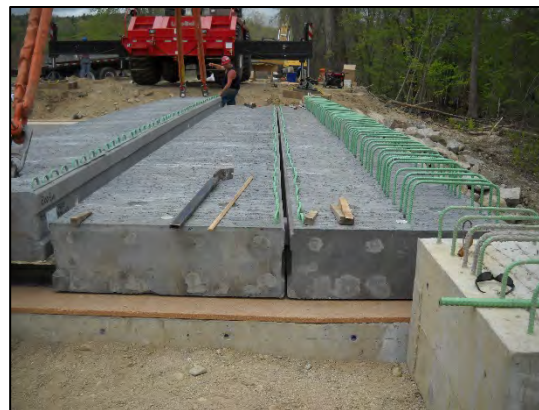
Alternative II Rehabilitation with Prestressed Precast Concrete Deck Beams over Arch
