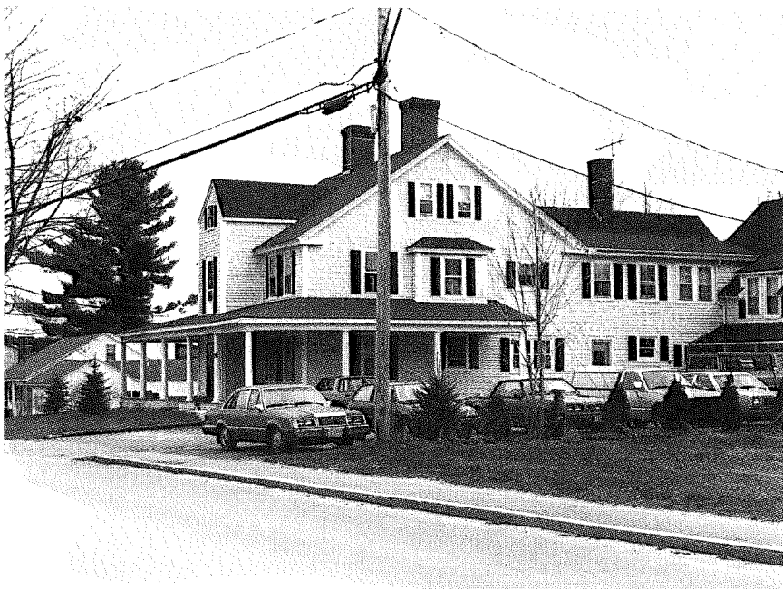
5-14 The Willard, later the Red Mill Inn, Stratton Road. Amos Stickney built this house soon after the Revolution. Later it was the residence of Perkins Bigelow and John Fox, and at one time it was owned by Susan Clay, the benefactress of the library. Bigelow (1791-1877) was one of the first in the town to take in summer boarders. The Willard was established as a hotel with 25 rooms in 1919 and continued in business into the 1940s. The elm tree to the left came down in the 1938 hurricane. The tower, porch and probably the back ell were all added over the years. Hotels and boarding houses catering to summer and later winter visitors were scattered throughout the town and to be successful didn't necessarily require extensive grounds or dramatic views of Monadnock. 1920s.
