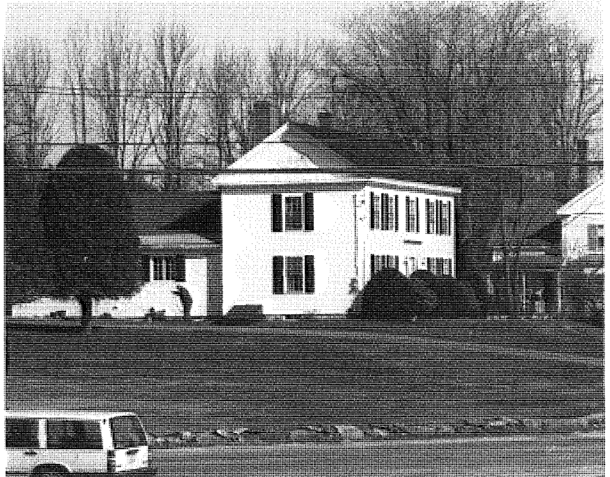
4-4 Sally Prescott House, 119 North Street. This house was probably built by William Hodge in the early 1800s. In 1823 he started a lead mill which continued operations into the present century. Hodge died in 1825 and his widow, Sally, married Benjamin Prescott, Jr. The house was later owned by G. S. Emery and John T. Crowe. In the earlier view the back ell suggests that the house might have started off as a one-story cape, the front two-story "main house" being added later. The entrance porch has disappeared as have the tall front-yard elms and the fencing. The earlier photograph was taken before School Street (now Goodnow Street) was extended across Main Street in 1874. Pre-1874.
