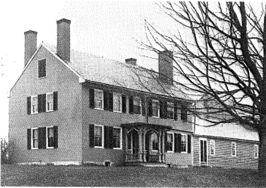
4-8 Following the fashion of the time the house was modernized and "Victorianized." The brick was painted gray, the original small-paned windows gave way to the latest "two-over-two" sash, a slate roof replaced the wood shingles and an elaborate Italianate entrance porch was added. The maples in the front yard were probably planted when the house was built in 1830: traditionally, one represents the husband, one the wife. (Sad to say, both of these maple veterans have succumbed since the modern photograph was taken.) The next stylistic transformation took place probably in the 1930s with the addition of a Colonial Revival porch and the change in paint color to white. Also, the barn was apparently thought to have outlived its usefulness and was moved to the Sawyer Farm on Turnpike Road where it was incorporated into the main barn complex still used today. Around 1980 a new though smaller barn was built but in a slightly different location. Ca. 1890s.
