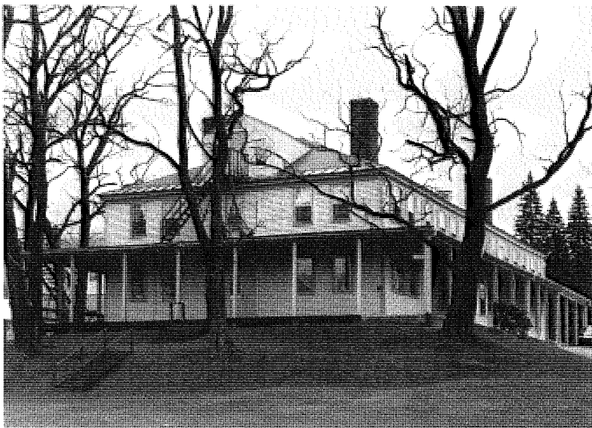
5-12 The Ark, Dublin Road. A view from the south shows some alterations to the porch and a dormer added to the hip roof, but unlike many other long-lived structures the basic massing of The Ark has remained. Expansion occurred more in the form of a series of separate cabins and annexes scattered throughout the extensive grounds. Between 1879 and 1882.
